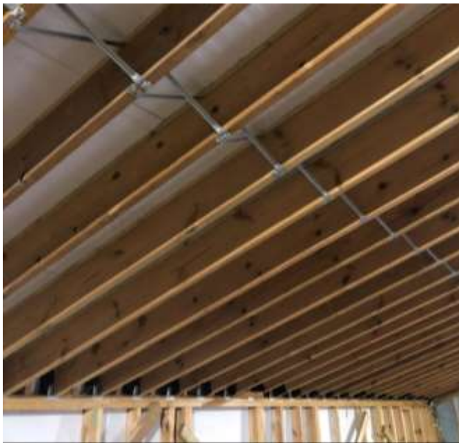
Photos of existing rafter detail.
