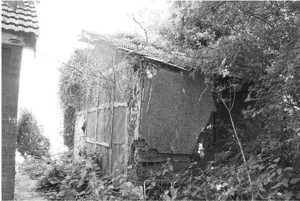
Photograph No. 05 – Building B2 is a dilapidated store offering ' negligible ' bat roost potential.
