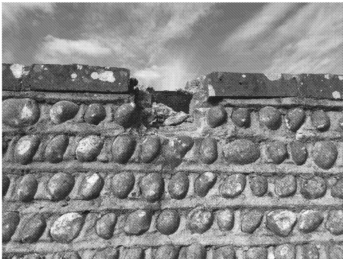
View on top of eastern boundary wall with central brick core visible
