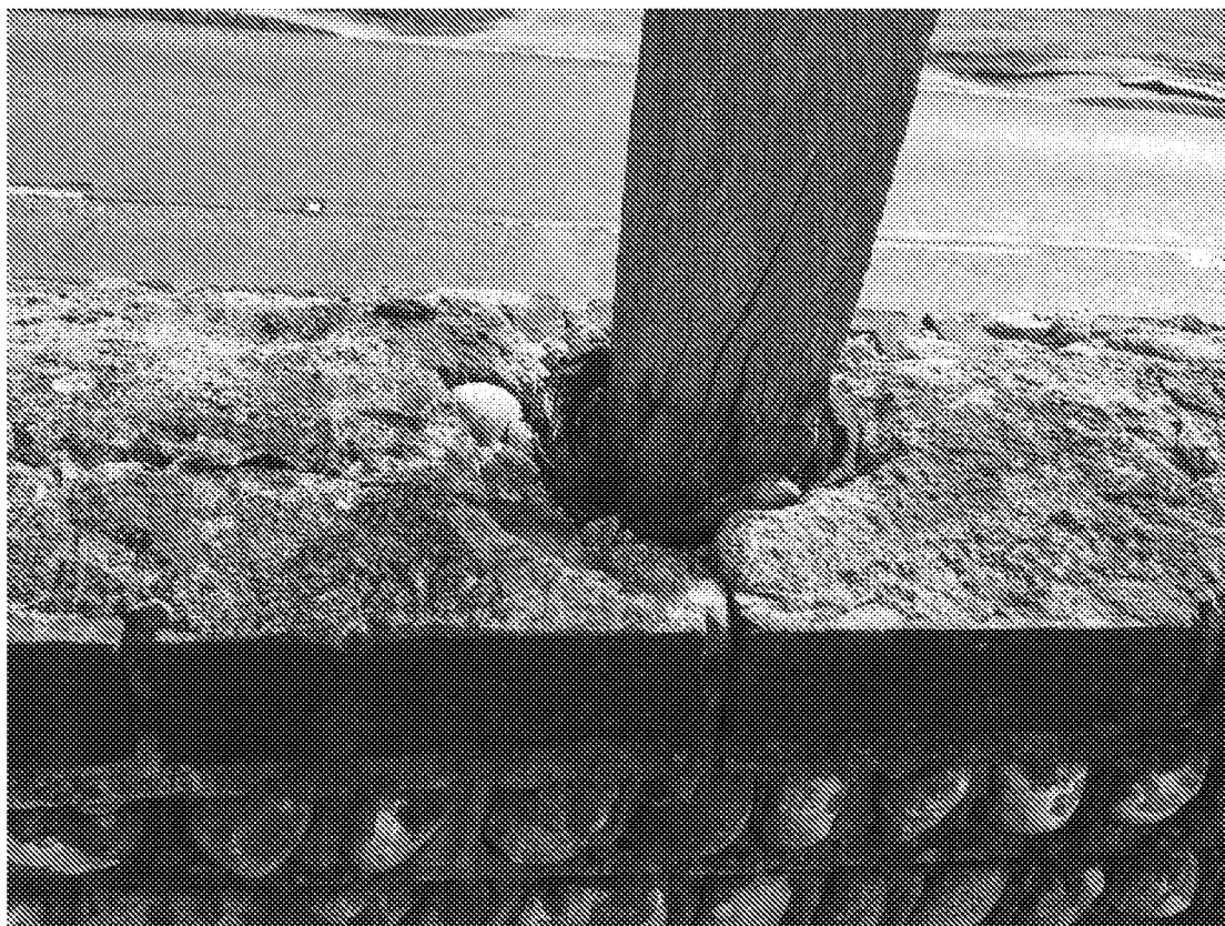
View on top of eastern boundary wall
