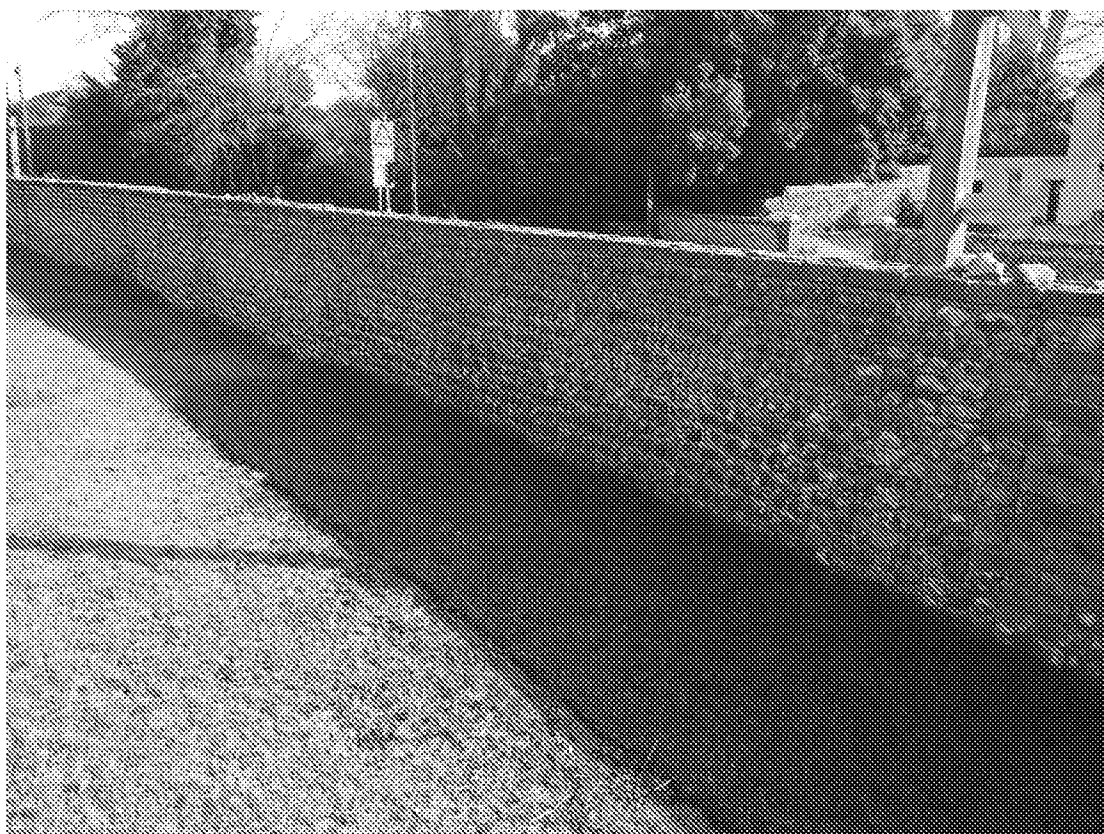
View on west face of eastern boundary wall
