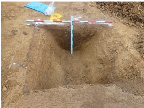
Plate 38: View of Section R , from the north-west
