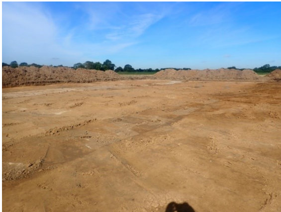
Plate 2: General view of the completed strip, map and record excavation area, from the north-east
