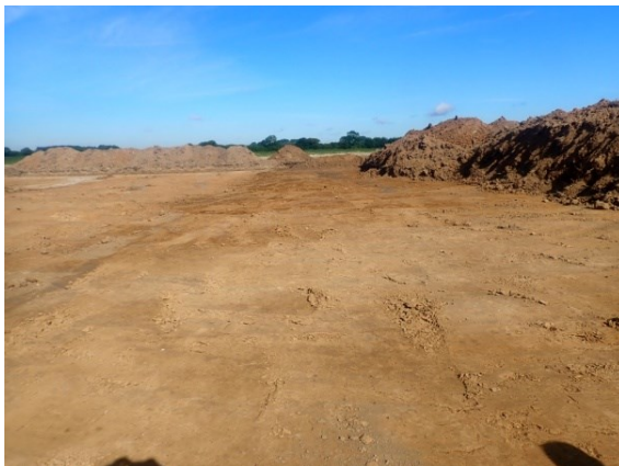
Plate 3: General view of the completed strip, map and record excavation area, from the south-east
