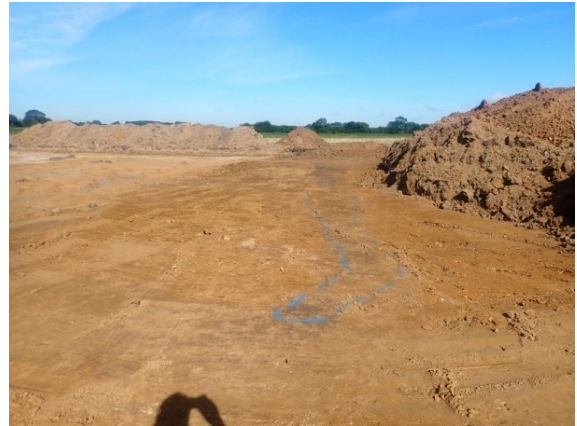
Plate 4: General view of the completed strip, map and record excavation area, from the south-east
