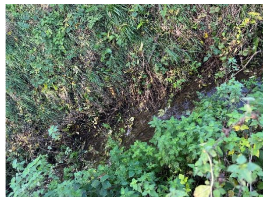
Section of ditch, Ryebank Rife, running along the western boundary of the site.
