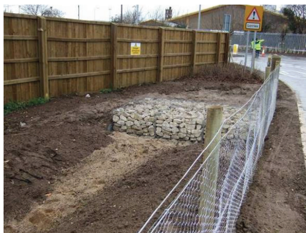
Gabion inlet shortly after construction (see diagram above)
