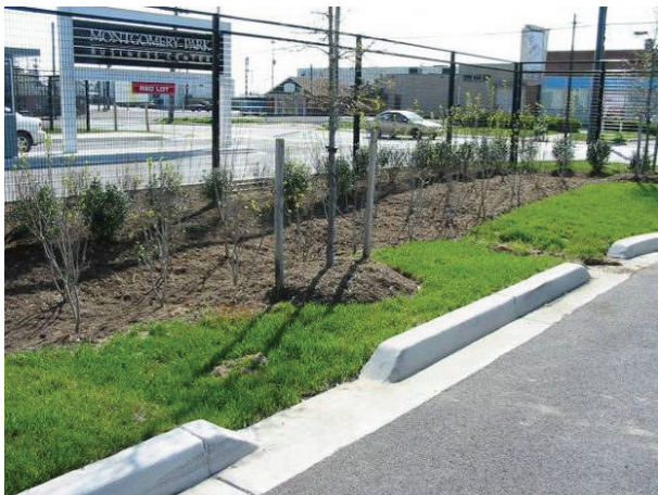
Dropped kerb inlet to rain garden
