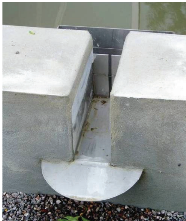
Slot weir outlet with steel plate to disperse water and debris guard behind
