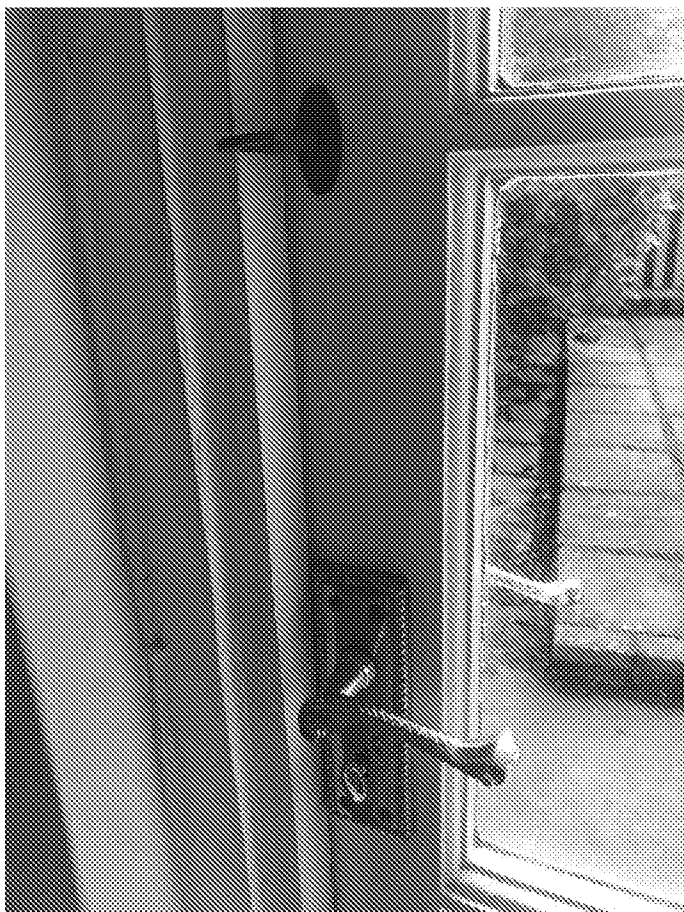
Figure 5 – Existing door surface bolt
