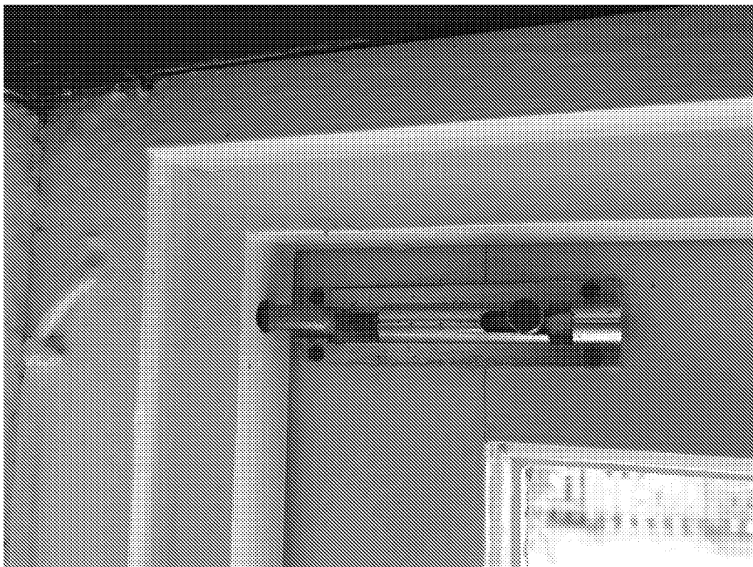
Figure 5 – Existing door surface bolt
