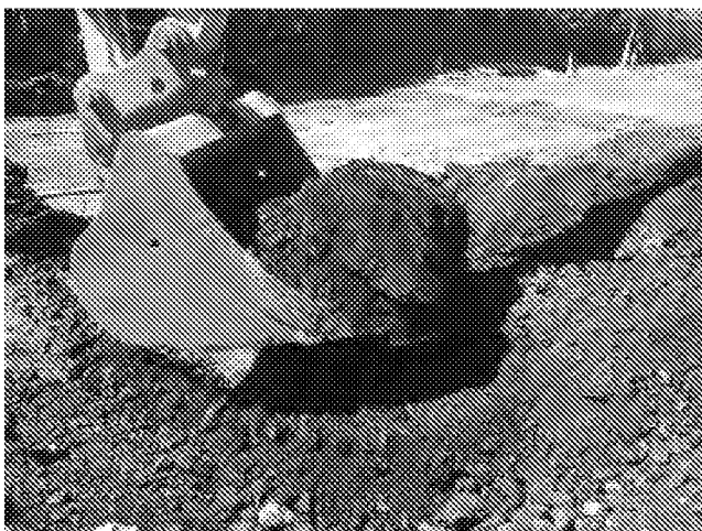
Segregating soils associated with TP07
