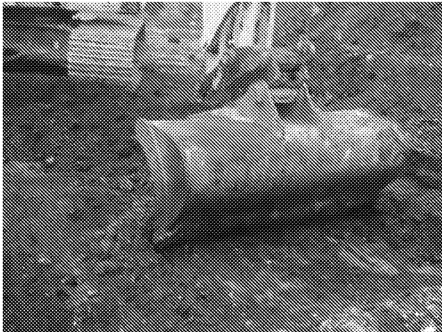
Segregating ashy soils associated with TP04 and SFTP04
