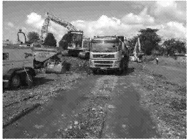
Loading away non-hazardous soils
