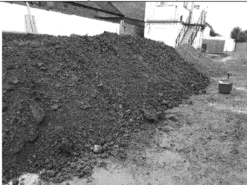
Stockpiled natural soils from excavation for soakaway Plots 5 to 8
