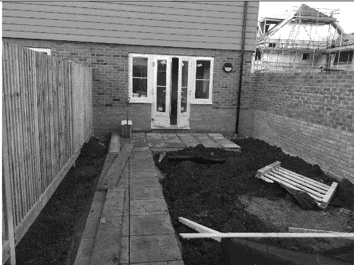
Topsoil to Plot 19
