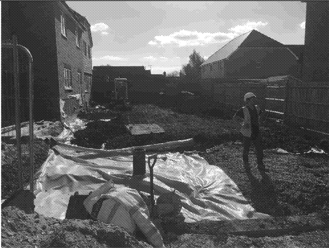
View South across Plots 5 to 8 during subsoil placement
