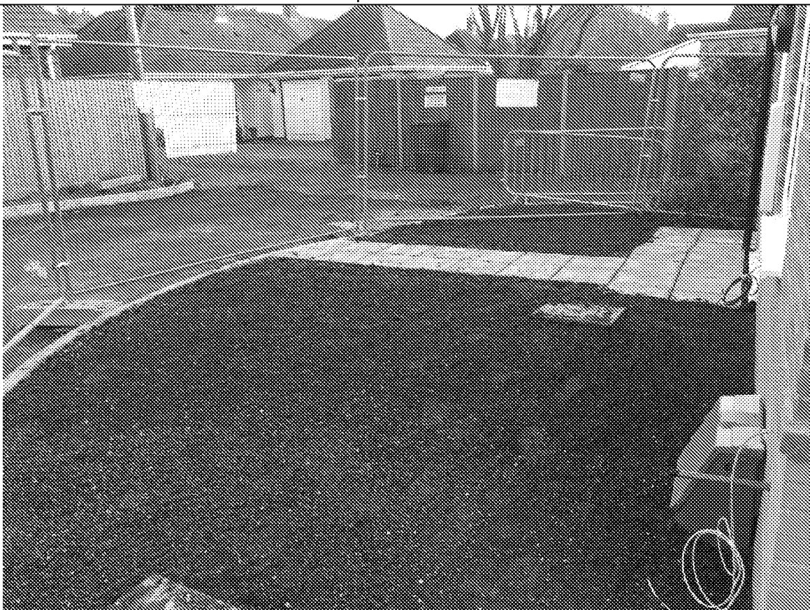
Topsoil to Plot 20 (Front)
