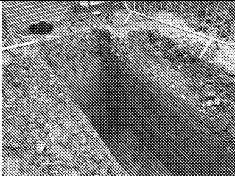
View south along excavation for soakaway Plots 5 to 8
