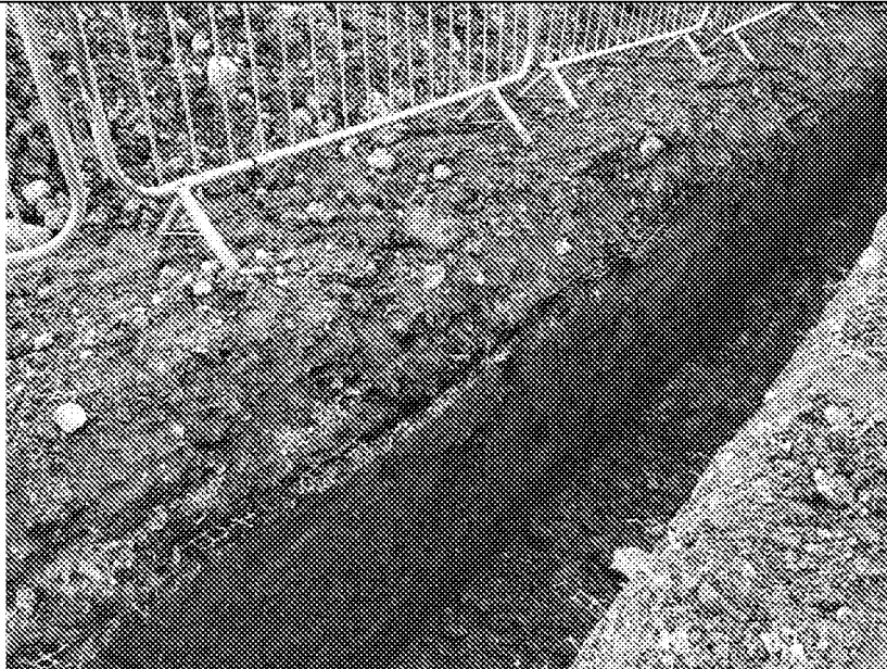
View north along excavation for soakaway Plots 5 to 8
