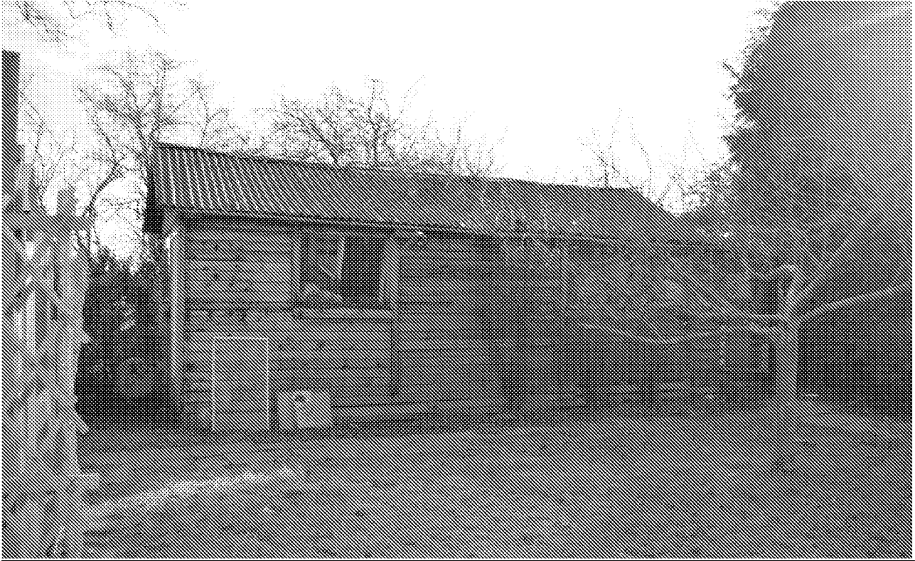
Fig 3. Photograph of the existing outbuilding that the proposal is intended to replace
