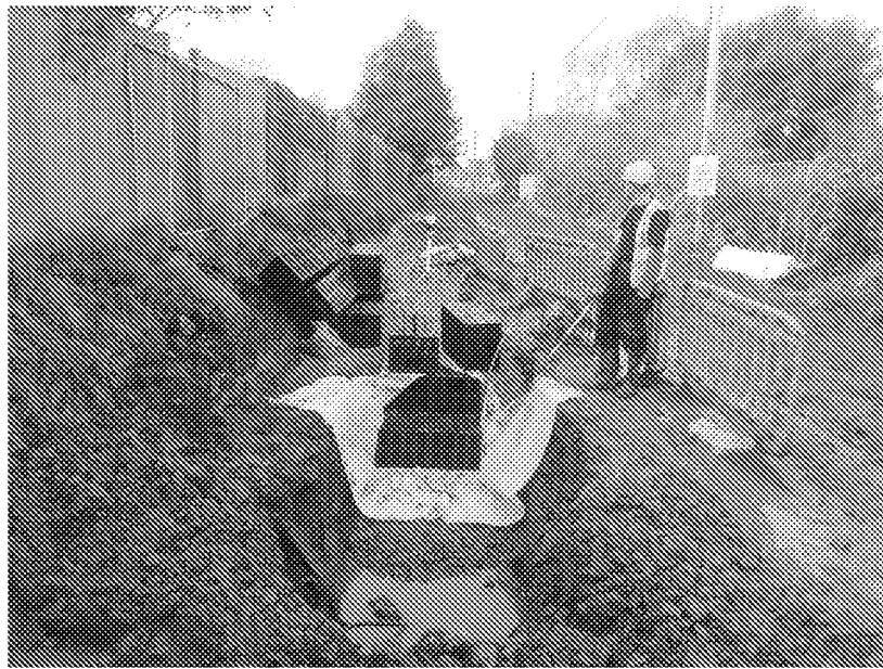
Figure 6: Photograph Showing the Geocellular Crates Underlain by Small Stone Aggregate
