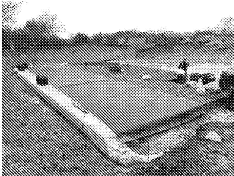
Figure 12: Photograph Showing the Geocellular Crates Wrapped in Impermeable Geomembrane
