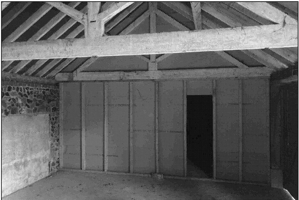
Photograph 4. The interior of the barn.
