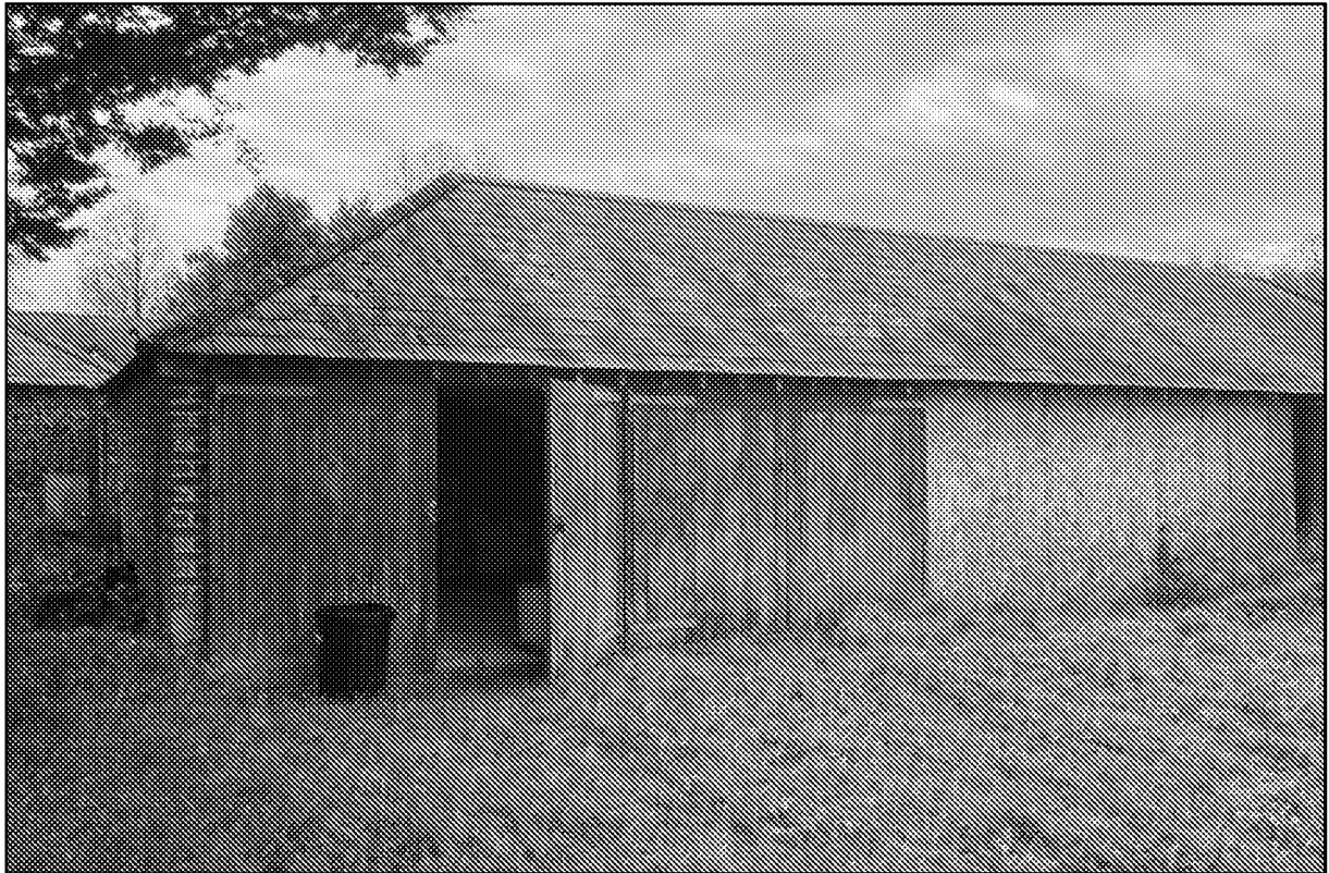
Photograph 1. The northern elevation of North Barn, Flansham.
