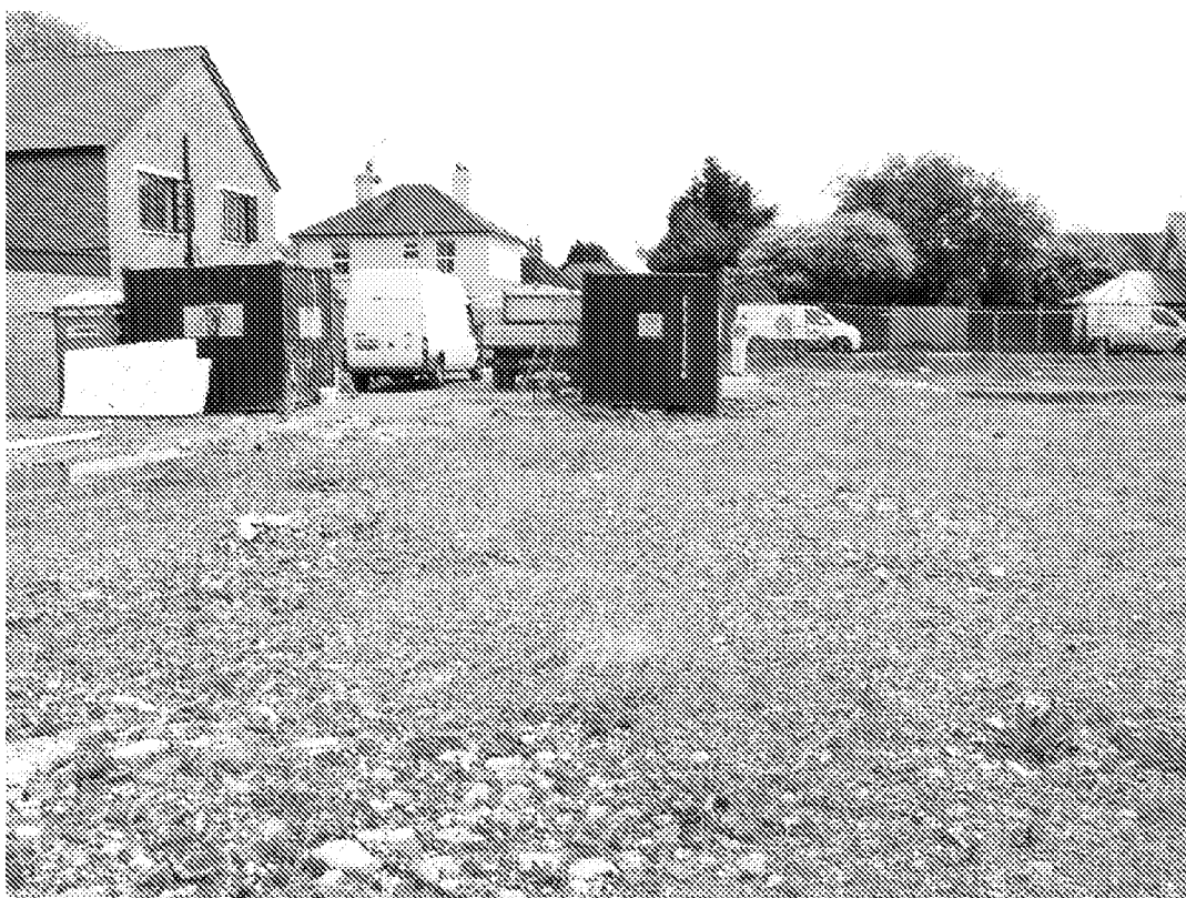
Figure 2. Bare ground (J4) - area of hard standing to support portacabins.
