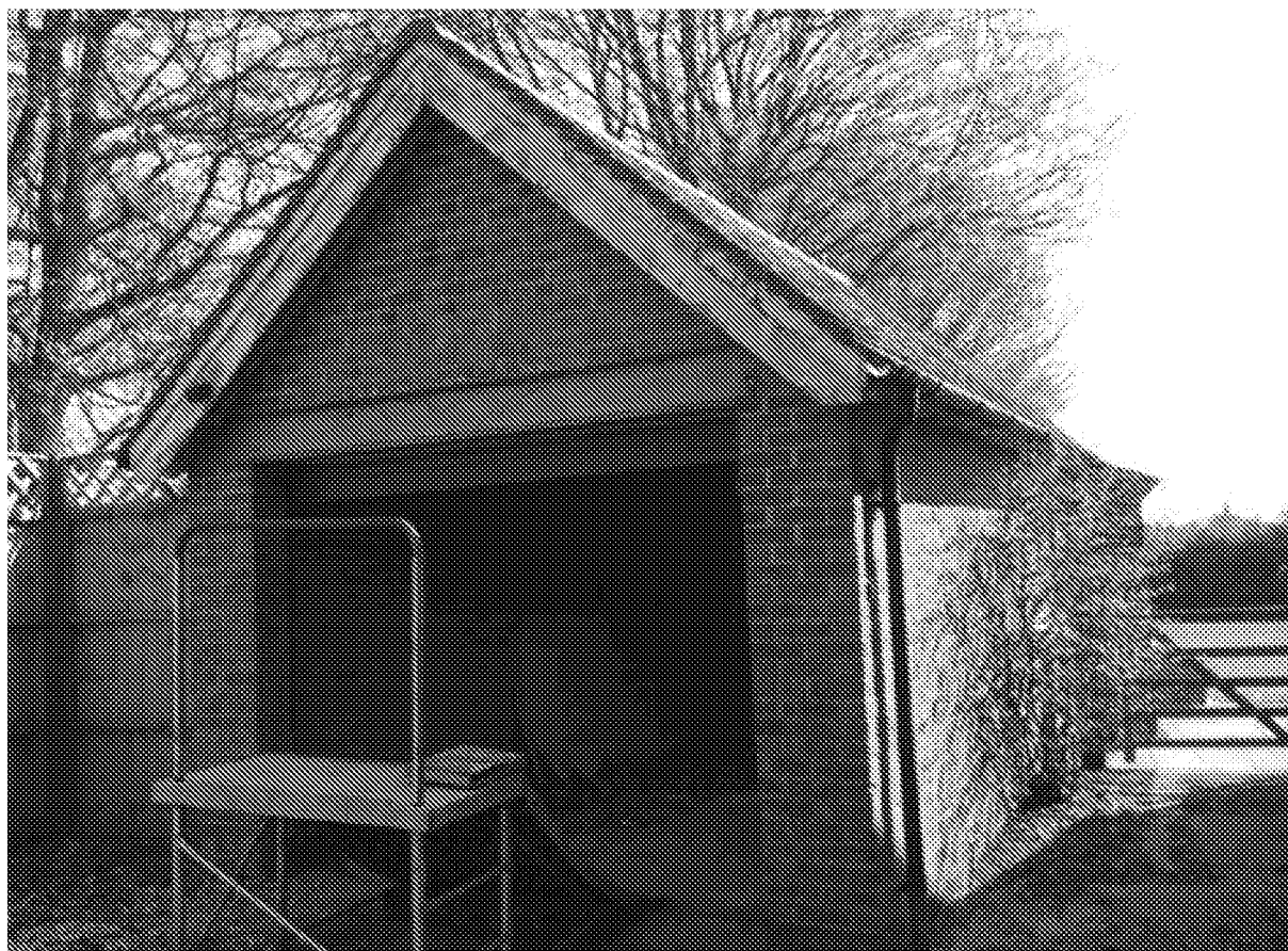
Figure 16. Brick walled outhouse located to the north of the southern property.
