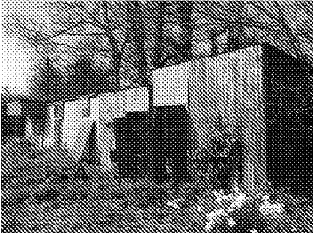
Figure 11. View of the dilapidated shed from the north east.
