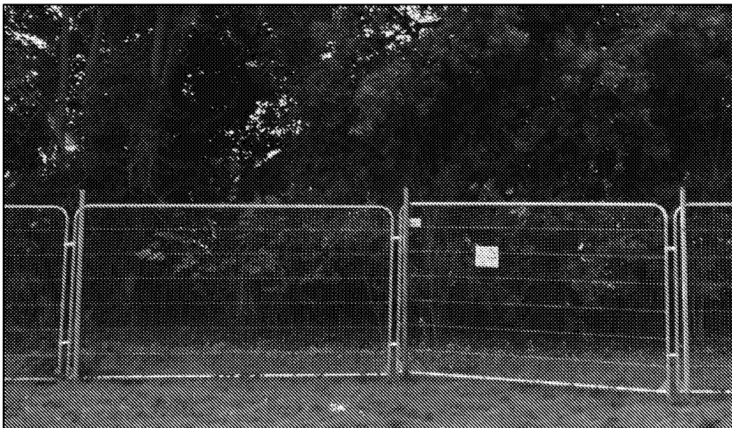
Weld-mesh panels on scaffold uprights
