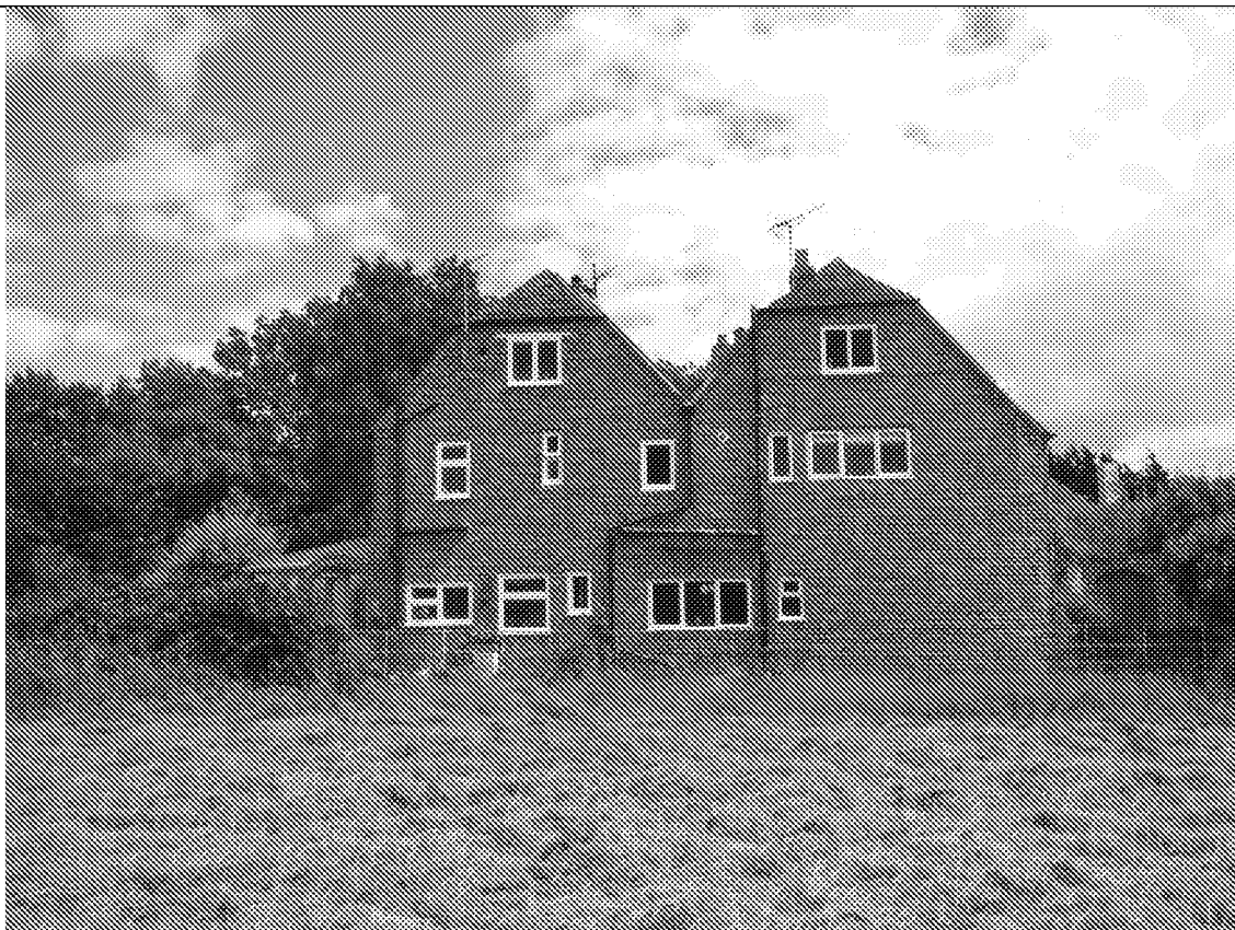
Plate 8: Laburnham Cottages' western elevation
