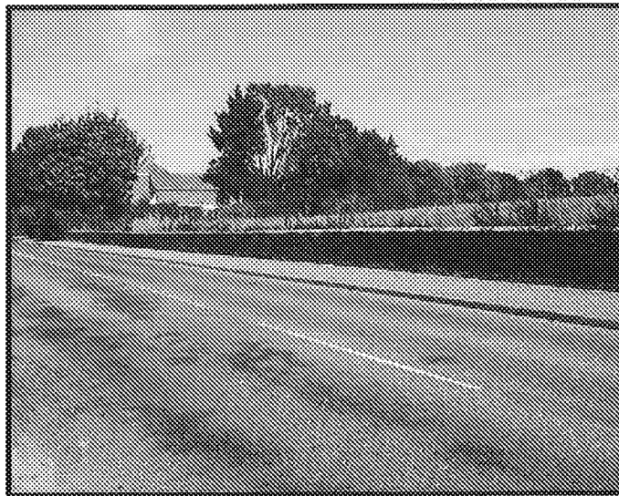
Road frontage, larger parcel
