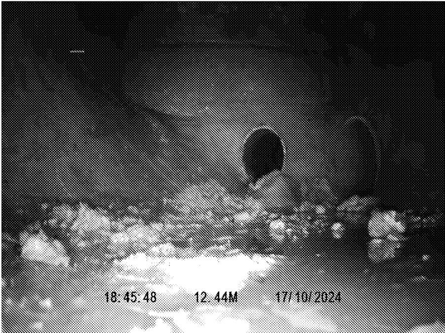
S63X_875222c7-28ab-42d3-8dc0-d5bee012671a_20241026_135131_327.jpg, 00:01:23, 12.44 m Finish node, manhole, reference: S63
