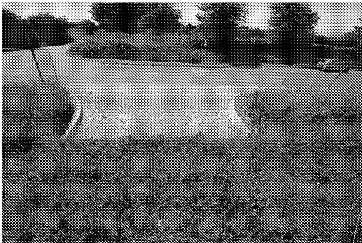
Frontage of Site following Reptile construction mitigation works (September 2020) and new access construction (photo, June 2021)
