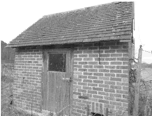
Building B3: External view, south-east aspect.
