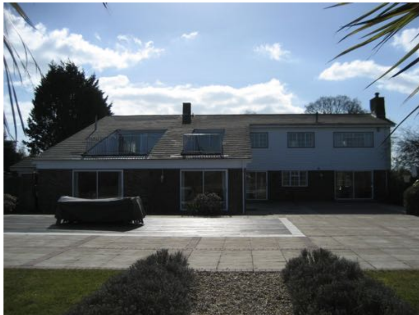
The Existing North (Rear) Elevation
