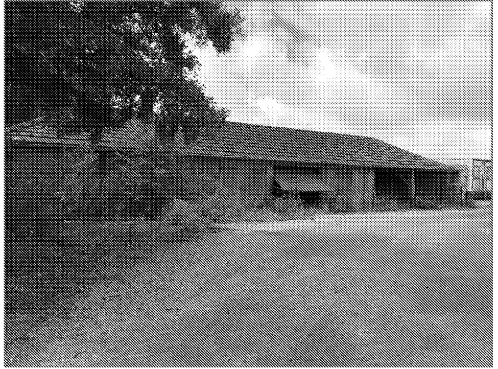
Plate 5 View of north-east elevation to the single-storey detached outbuilding that occupies the south-west corner of the subject site. Note that this building dates from the mid-19 th century with 20 th century alterations.
