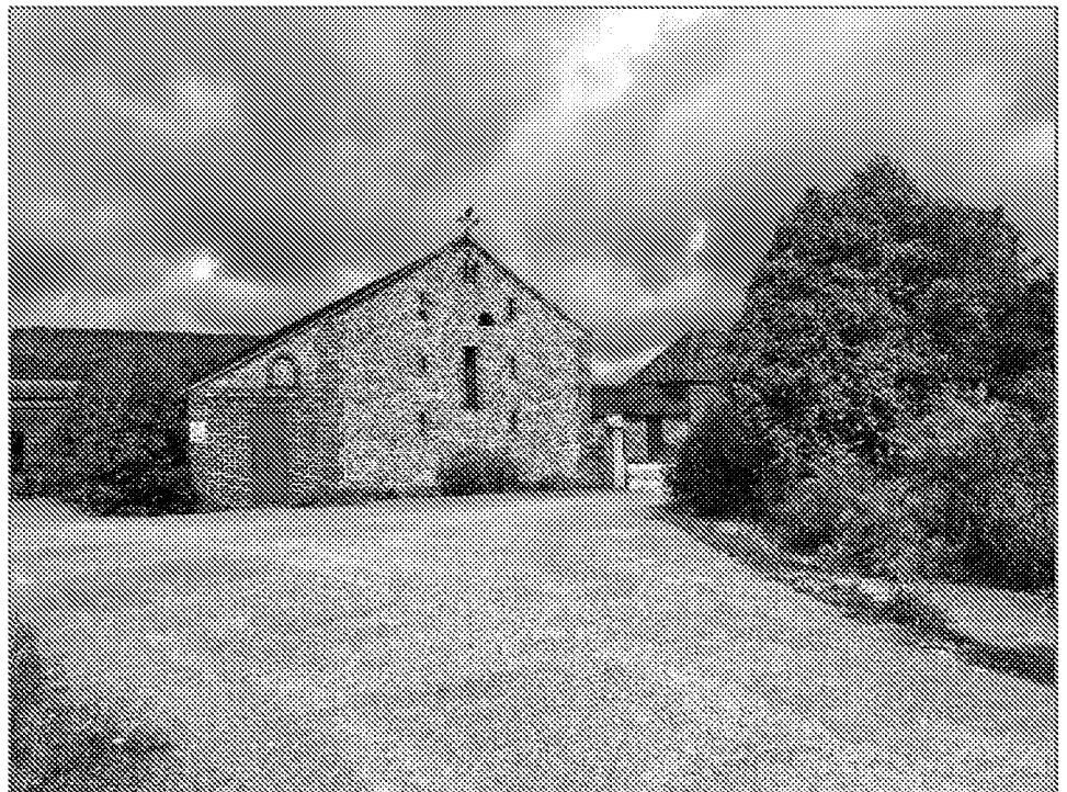
Plate 4 View of south-east elevation to the former barn occupying the southernmost part of the outbuildings group. Note that this structure dates from the mid-19 th century.
