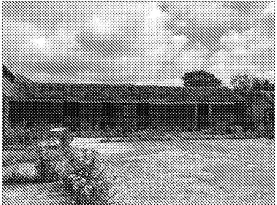
Plate 8 View of south-west elevation to outbuilding wing located in north-western part of subject site. Note that this wing forms the north-eastern part of the main U plan outbuilding group with its earlier fabric dating from the mid-19 th century. It has seen notable change during the 20 th century.
