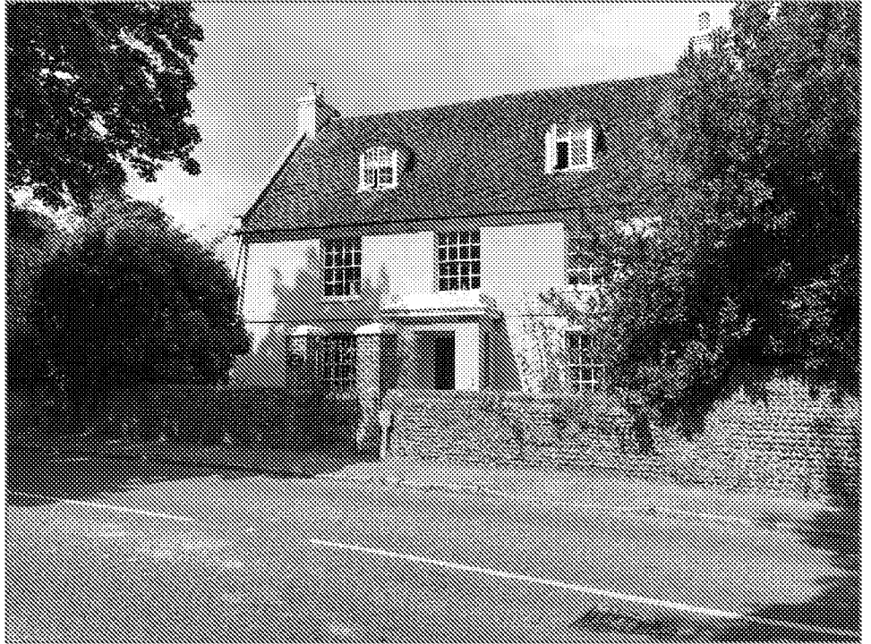
Plate 1 View of principal front (south-east facing) elevation to the Grade II listed Stakers Farmhouse. Note that this view is taken from North End Road.
