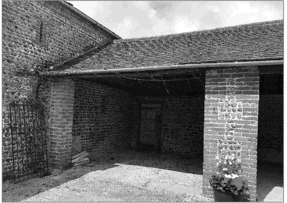
Plate 11 Part view of southernmost bay to the courtyard (south-east) elevation to the single-storey element that adjoins the two-storey barn (Barn 2).
