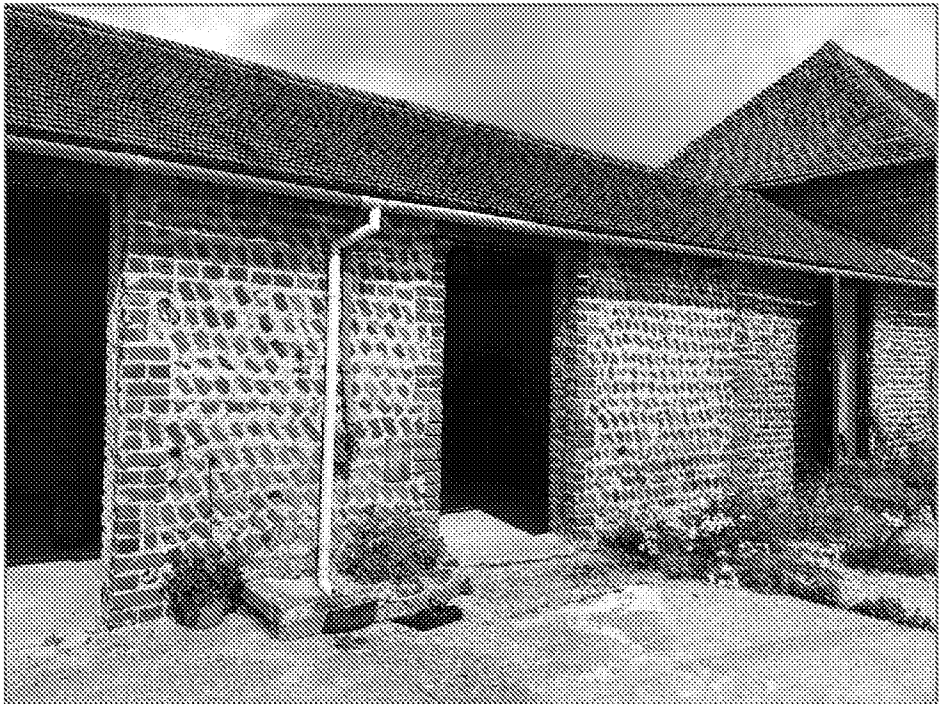
Plate 12 Part view of central bay to the courtyard (south-east) elevation to the single-storey element that sits between the two-storey barns. Note that the approved timber framed windows will be introduced to each of the existing openings. The proposal includes a number of changes to the approved fenestration.
