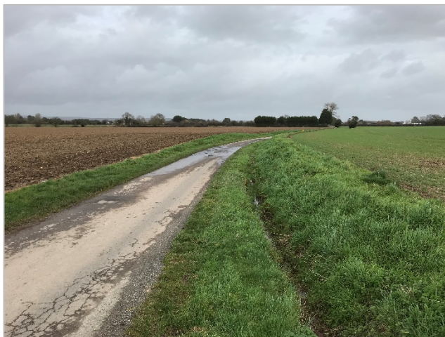
FACING NORTH ON DROVE LANE – NOTE: DITCH AND STEEP GRADIENT
