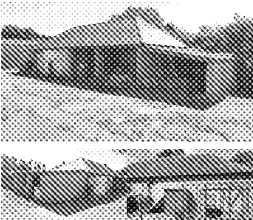
Fig 7-9. Existing Outbuilding (proposed to be converted to ancillary accommodation to main dwelling)
