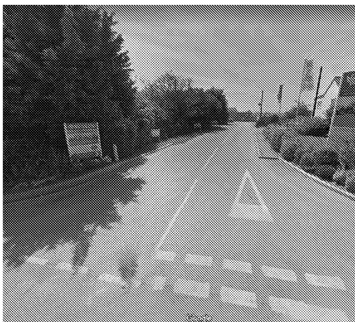
Figure 13: Existing Access to Nursery
