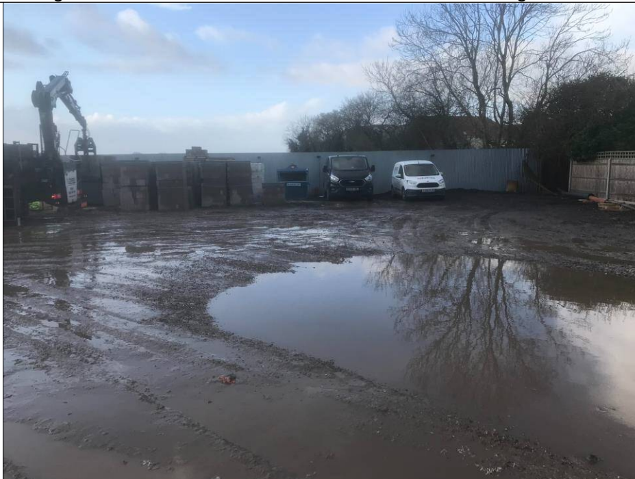
Looking south from access gate, towards south western corner of site.
