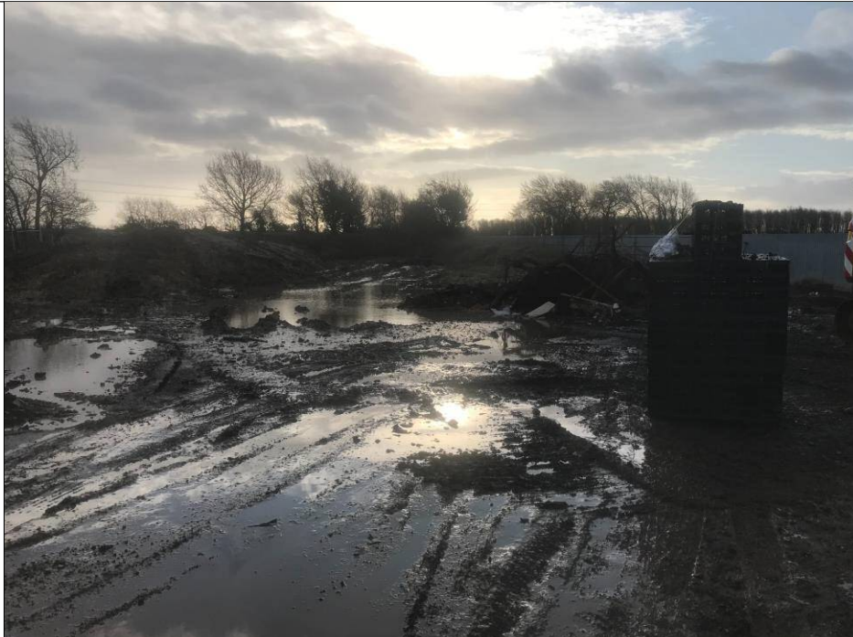
Looking toward the south eastern corner of the site from the access gate.
