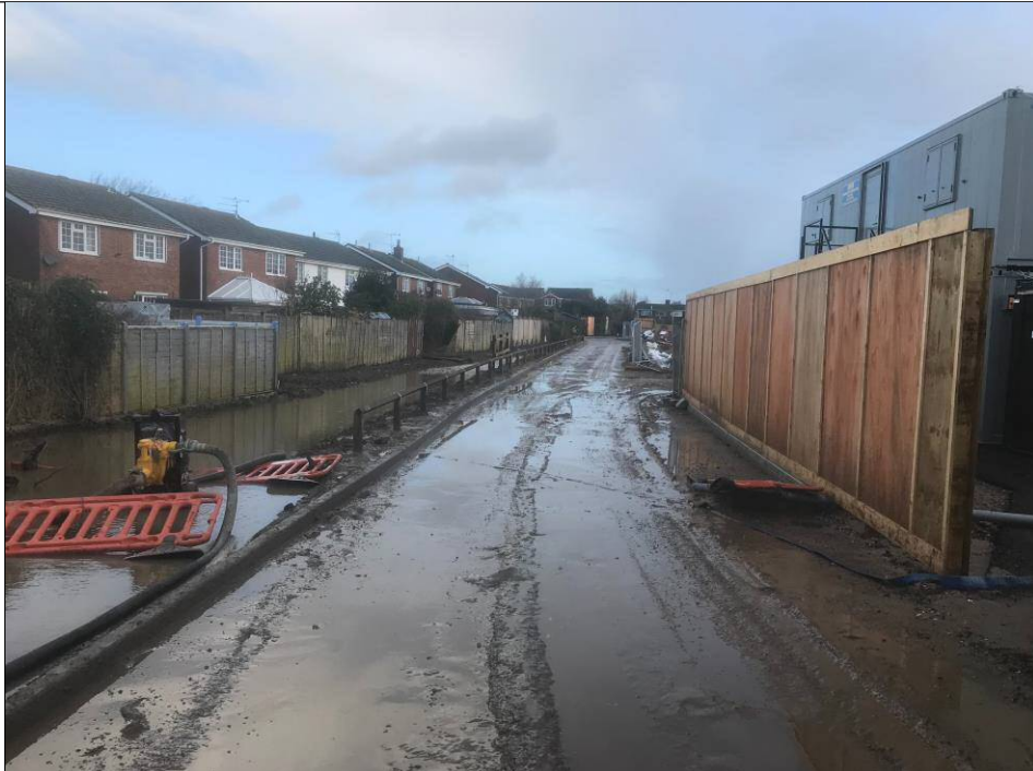
Looking east along northern site boundary at adjacent construction site
