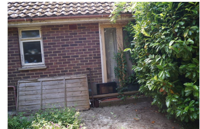
Windows/doors at Nyasa facing boundary
