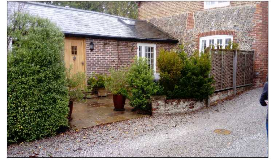
Photograph of existing fence
