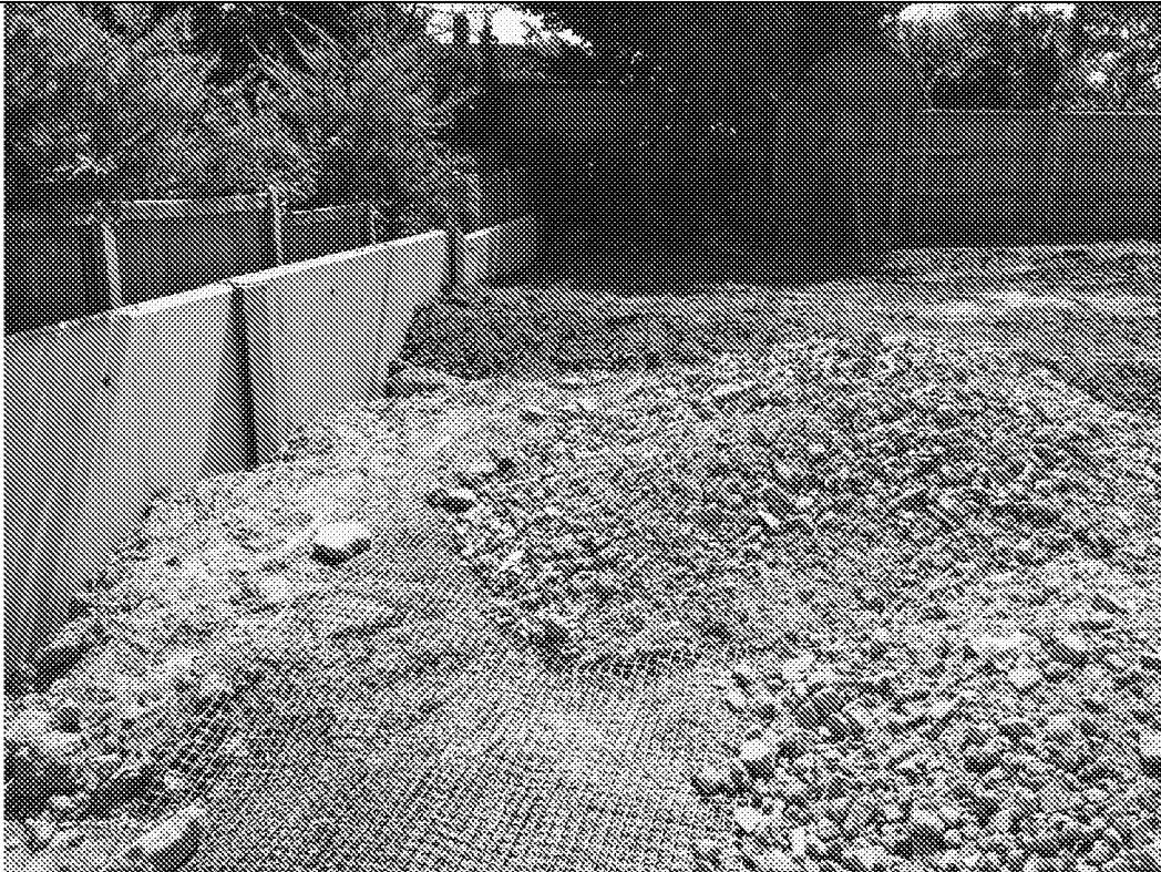
View south across Plot 16 showing sub soil placement
