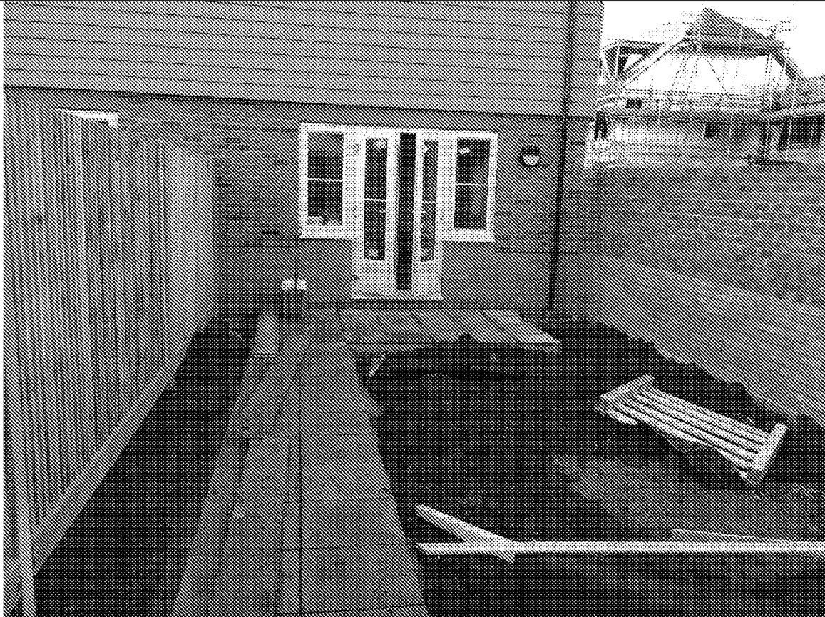
Topsoil to Plot 19
