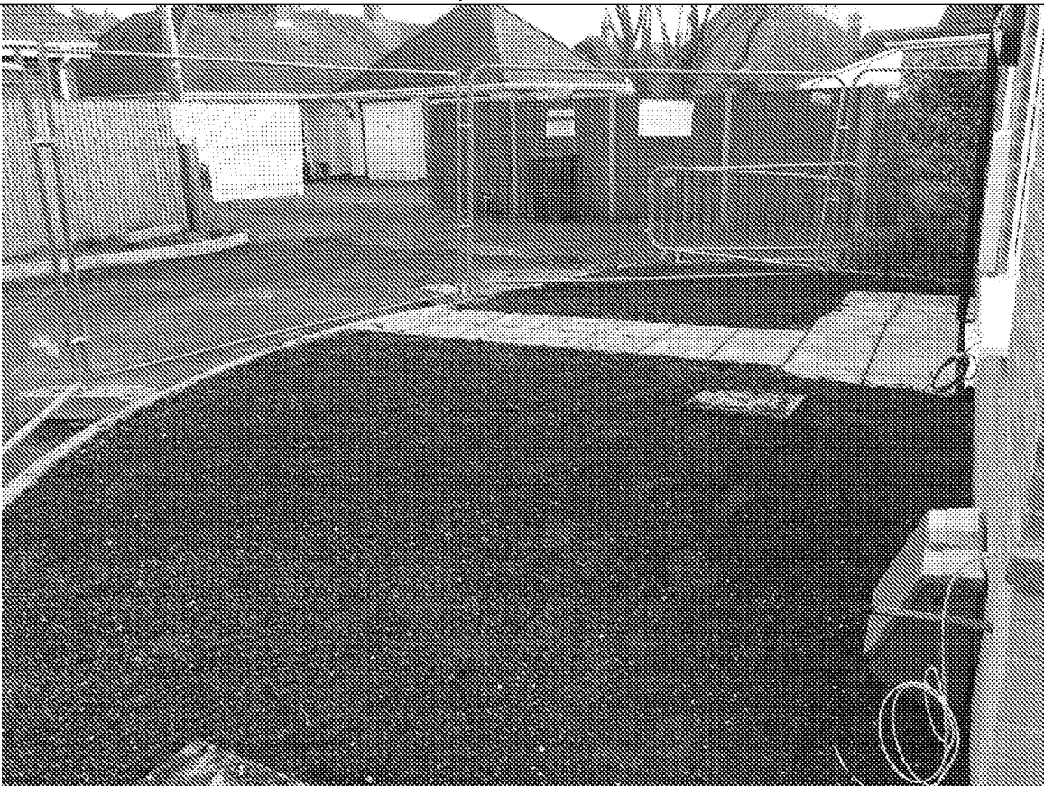
Topsoil to Plot 20 (Front)
