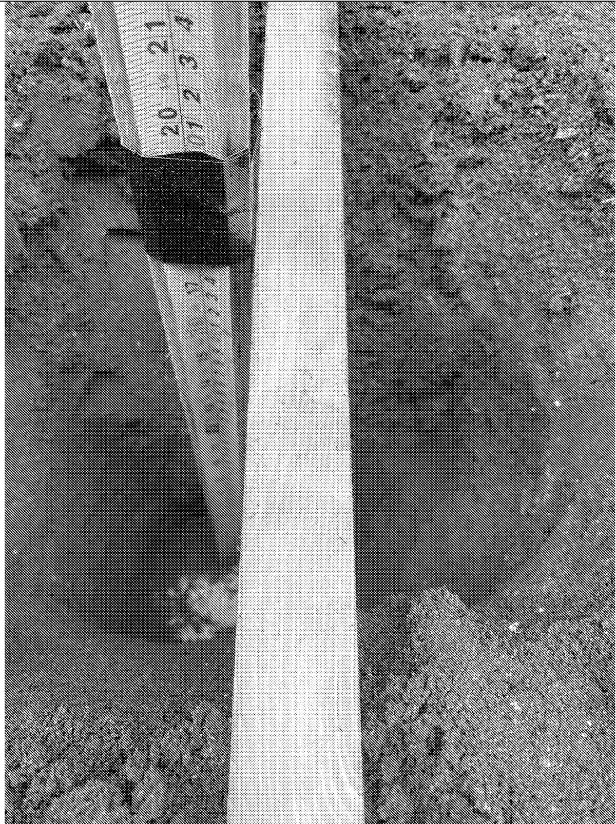
Photograph 3: View of trial hole rear garden confirming depth to base and cover > 450mm
