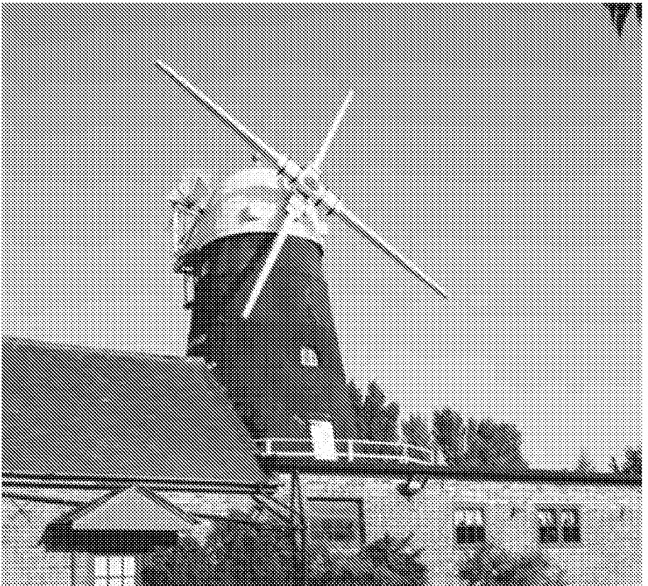
Figure 43: View of Barnham Windmill looking east
