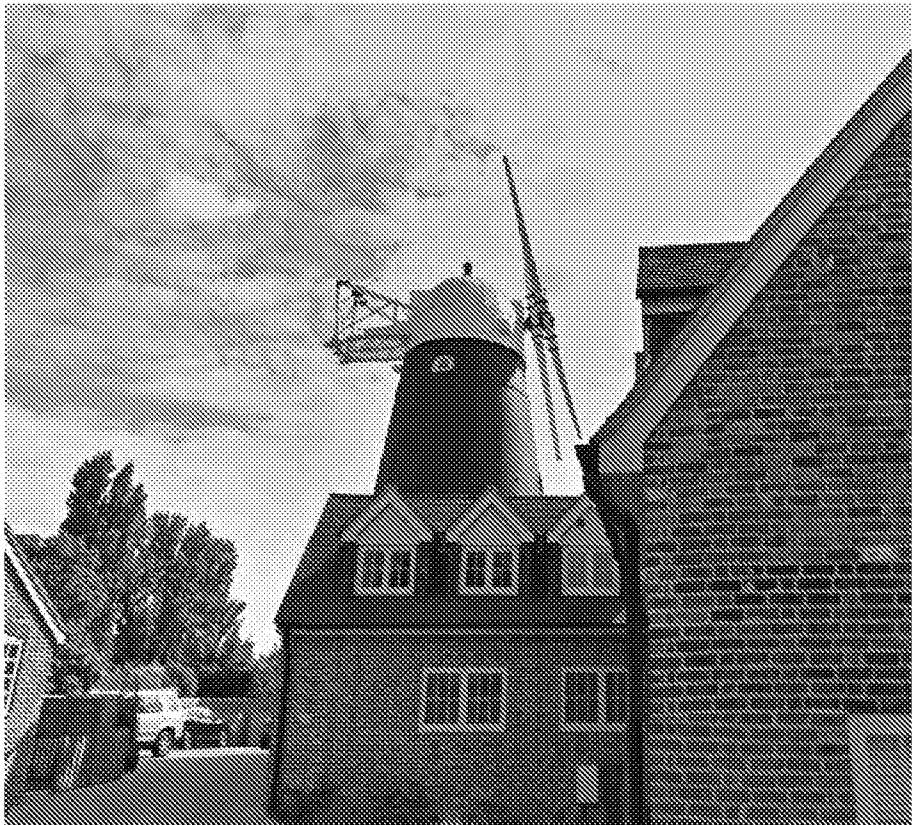
Figure 42: View of Barnham Windmill from Main Road looking south along Yapton Road
