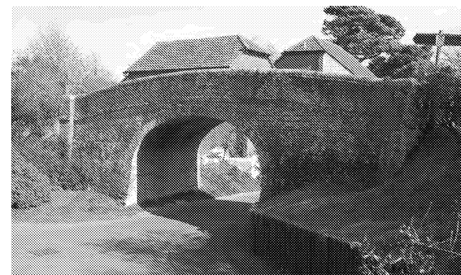
Figure 7: Bridge over what was once the course of the Portsmouth and Arundel Canal during the 19th century
