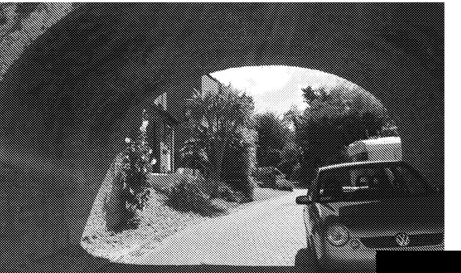
Figure 27: View eastward through the canal bridge, demonstrating how the setting had been eroded by the recent development
