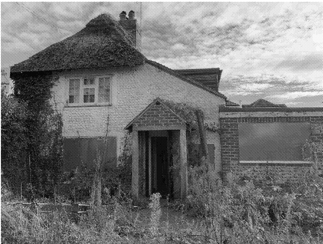
North elevation thatch:
