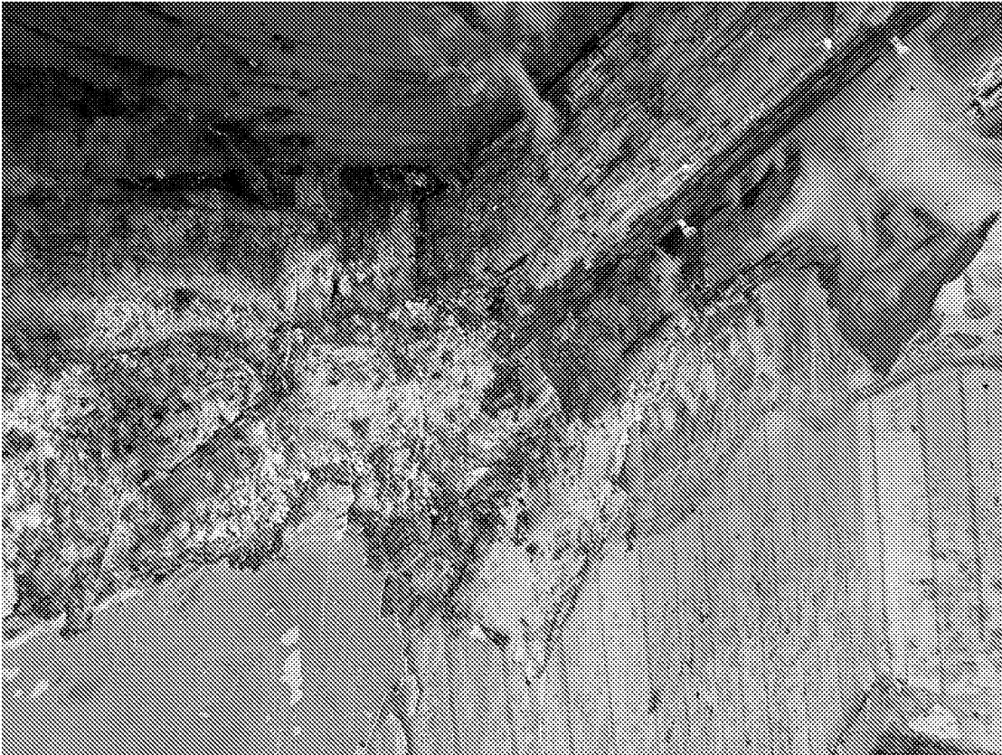
Side roof timber failure due to wet rot:
