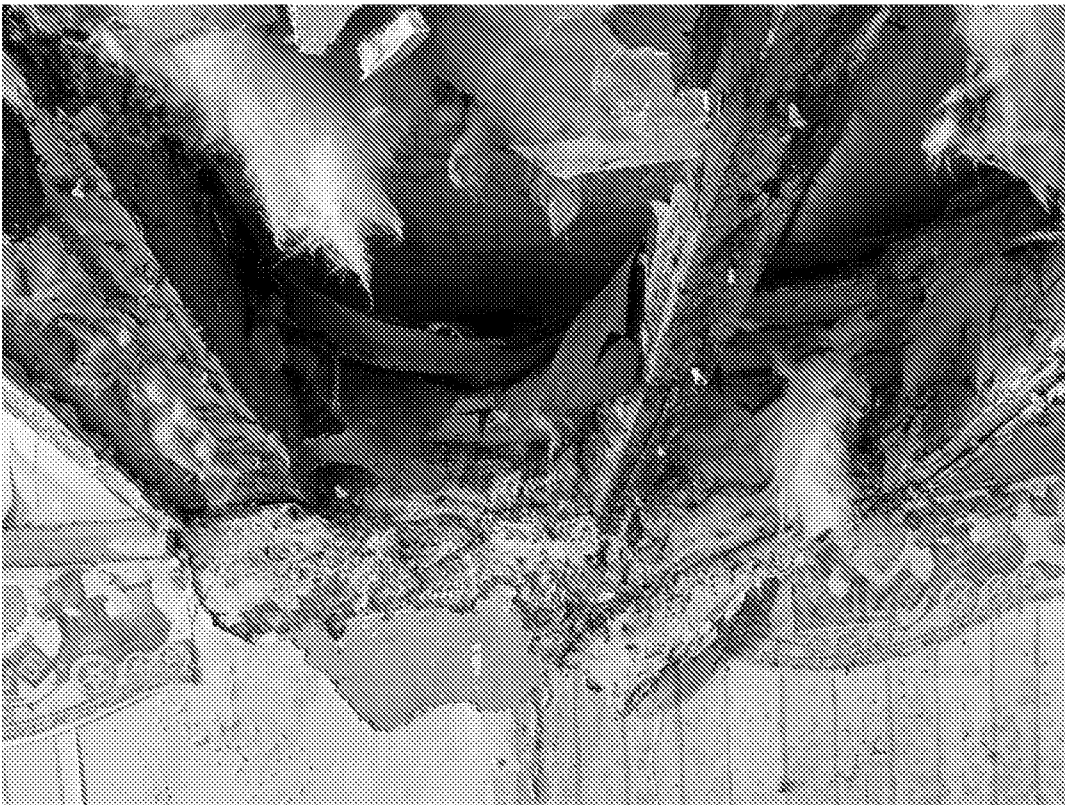
Side roof timber failure due to wet rot:
