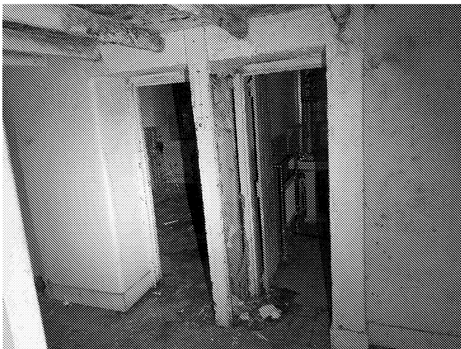
Fig A3 – Hall, showing beams.
