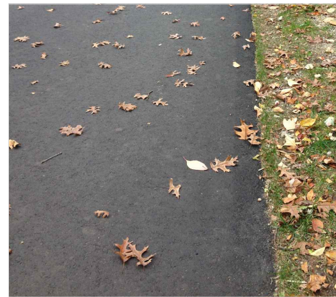
IMAGE 1 Pedestrian Tarmacadam surface finish
