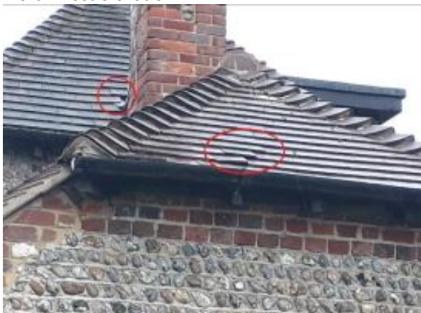
Raised tiles on north elevation
