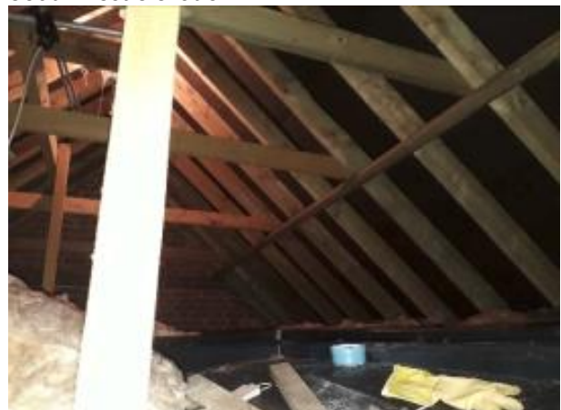
Roof void of main house
