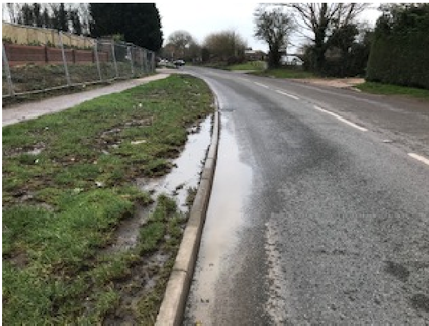
Figure 3: Ponding on the eastern channel on North End Road.
