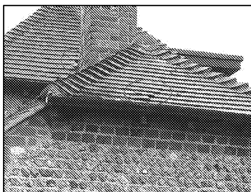
Figure 12: Raised tiles on main house
