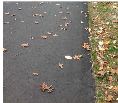
IMAGE 1 Pedestrian Tarmacadam surface finish
