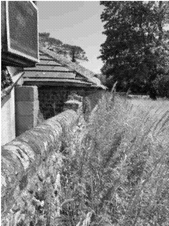
Building 5 – Front elevation showing the flint/brickwork end of the elevation and vertical crack
