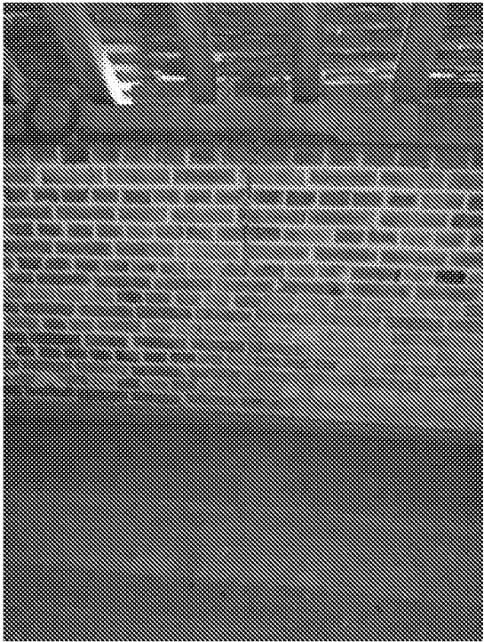
Building 2 – Loose/missing brickwork at low level
