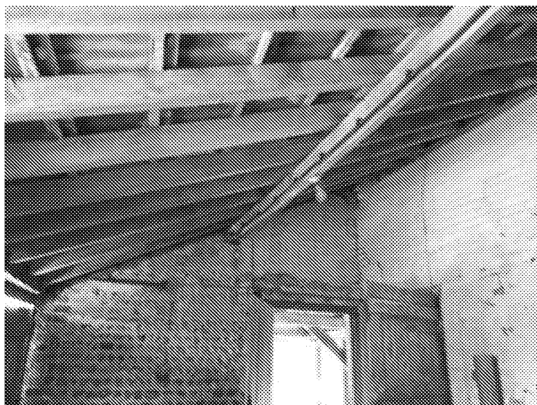
Building 2 – Single storey area with mono-pitched roof, showing diagonal cracking above doorway
