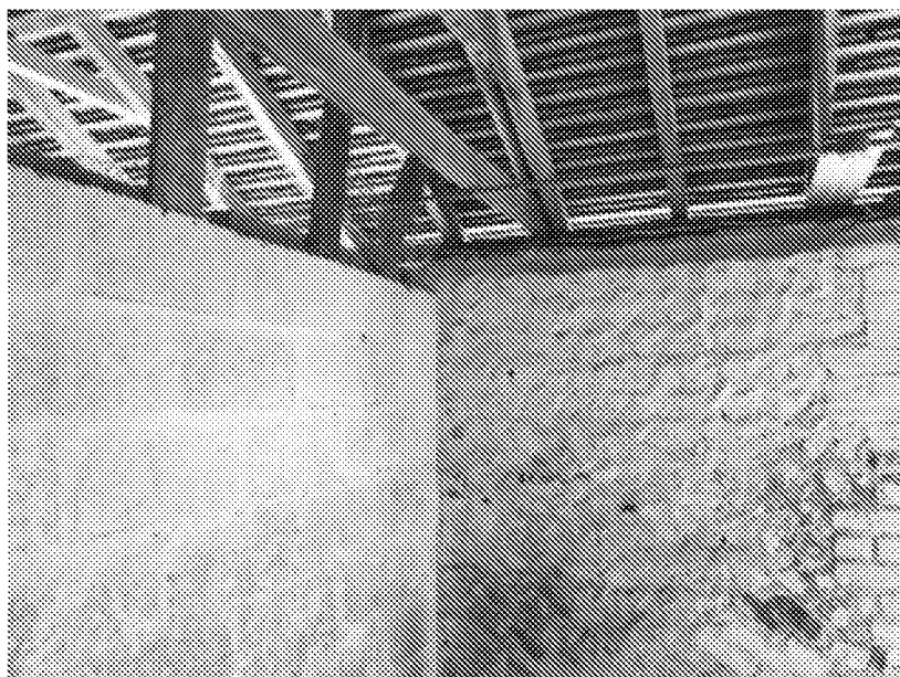
Building 3 – Timber roof trusses formed from rafters, ties, collars and purlins and room division wall
