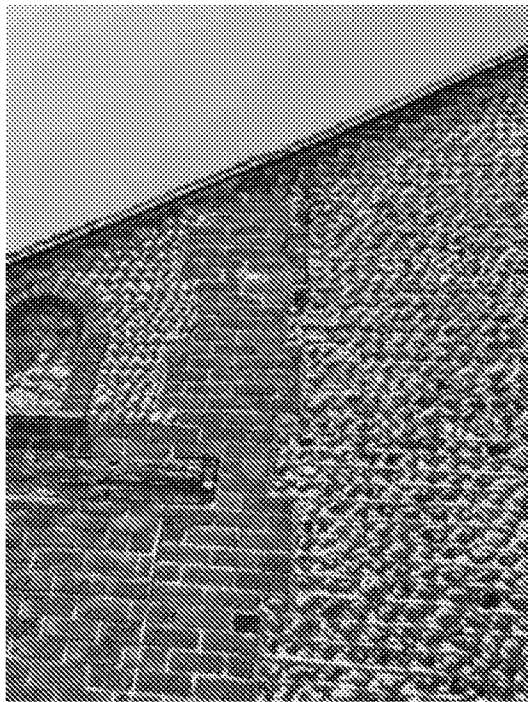
Building 4 – Cracking between flint and brickwork
