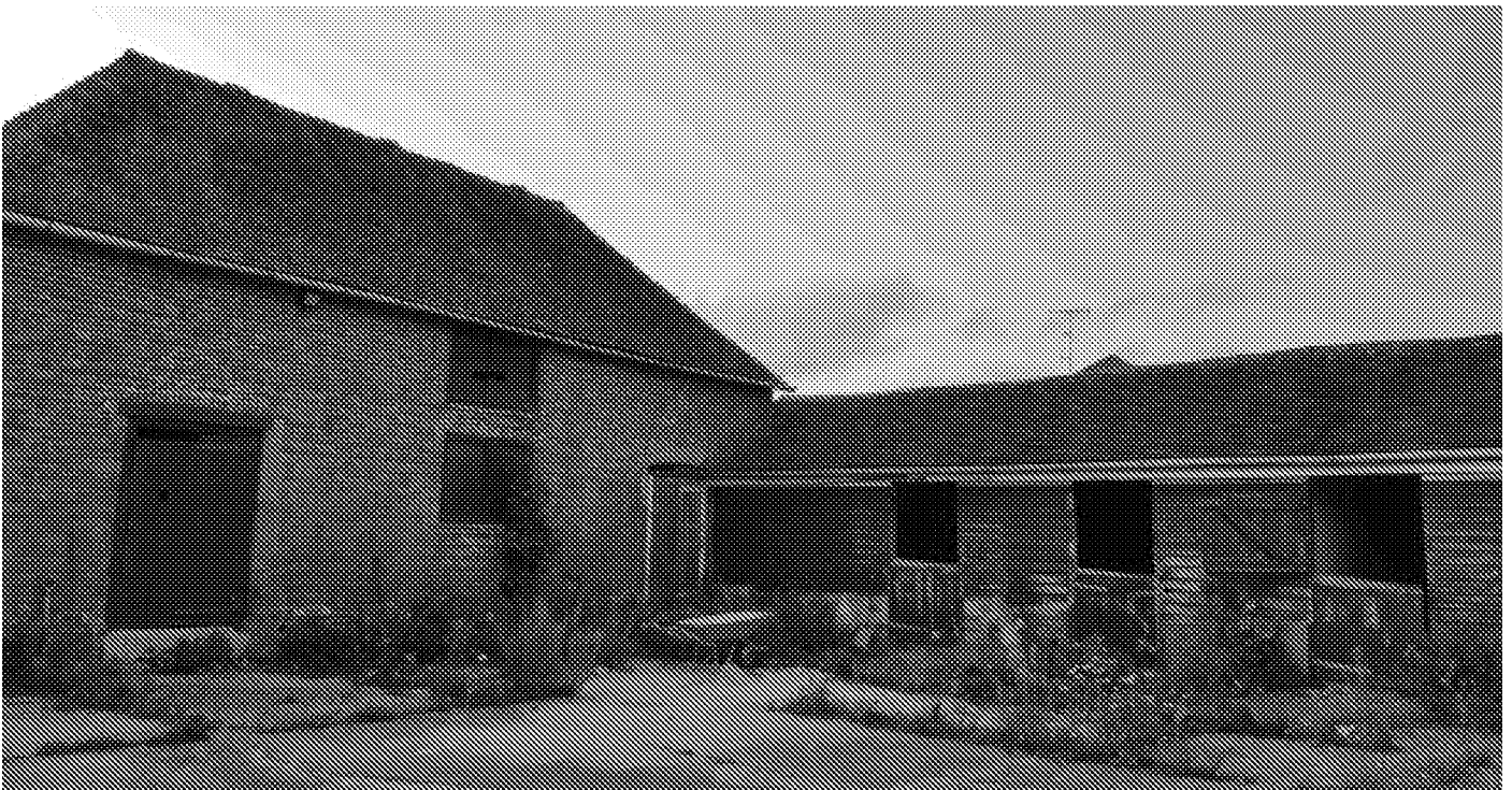
Photograph No. 2 - Building B3 (left) which supports a night roost / feeding perch of long-eared bats and Building B4 (right) which supports a day roost of common pipistrelle.
