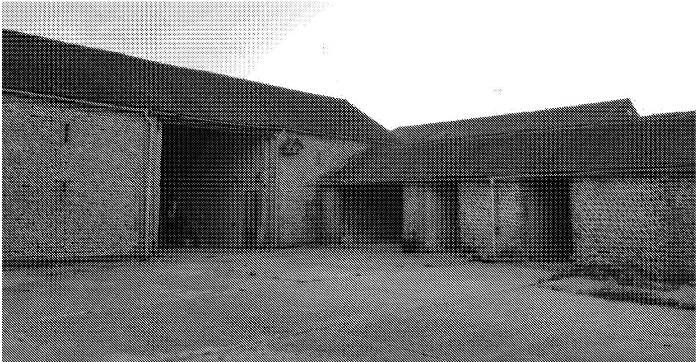
Photograph No. 1 - Buildings B1 (left) and B2 (right). Both buildings were subject to full bat surveys; no bat roost was found.
