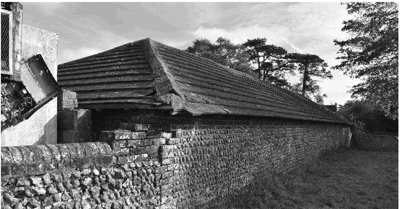
Photograph No. 8 - Building B6, heavy concrete tiles and open eaves with no signs of bats noted.
