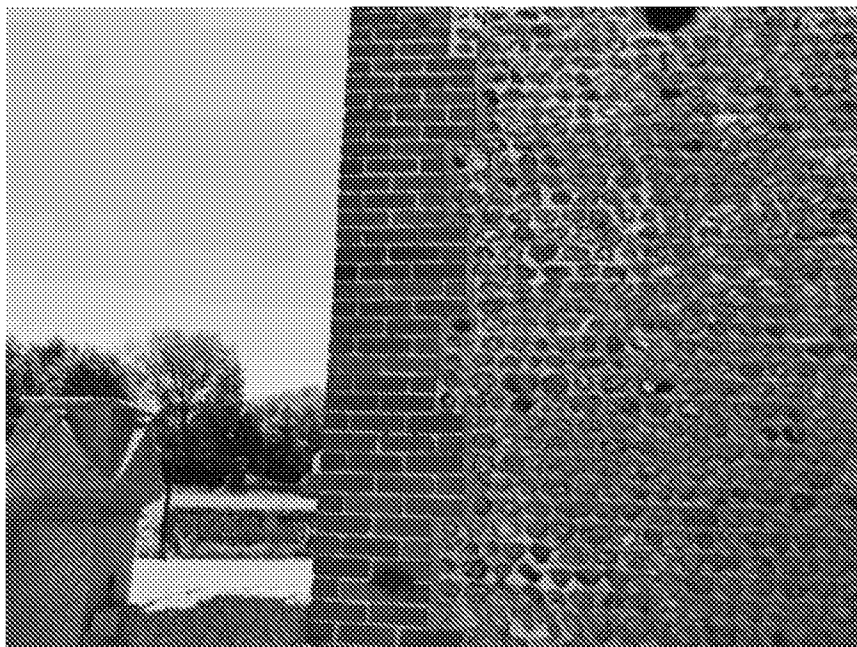
Building 4 – Cracking between flint and brickwork on corner
