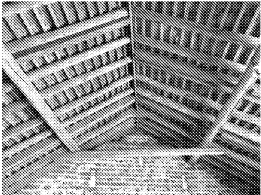
Building 1 – Roof rafters with purlins and one number collar/ties for lateral restraint
