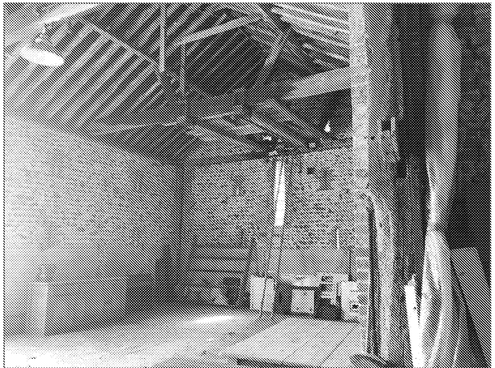
Plate 18 View of part interior to two-storey barn (part of Outbuilding 2). Note that this double height space will be retained.
