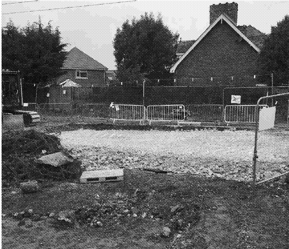
Figure 18: Imported clean stone used as backfill following asbestos removal works
