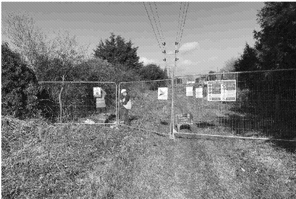
Figure 1: Heras fencing and site safety signage is installed
