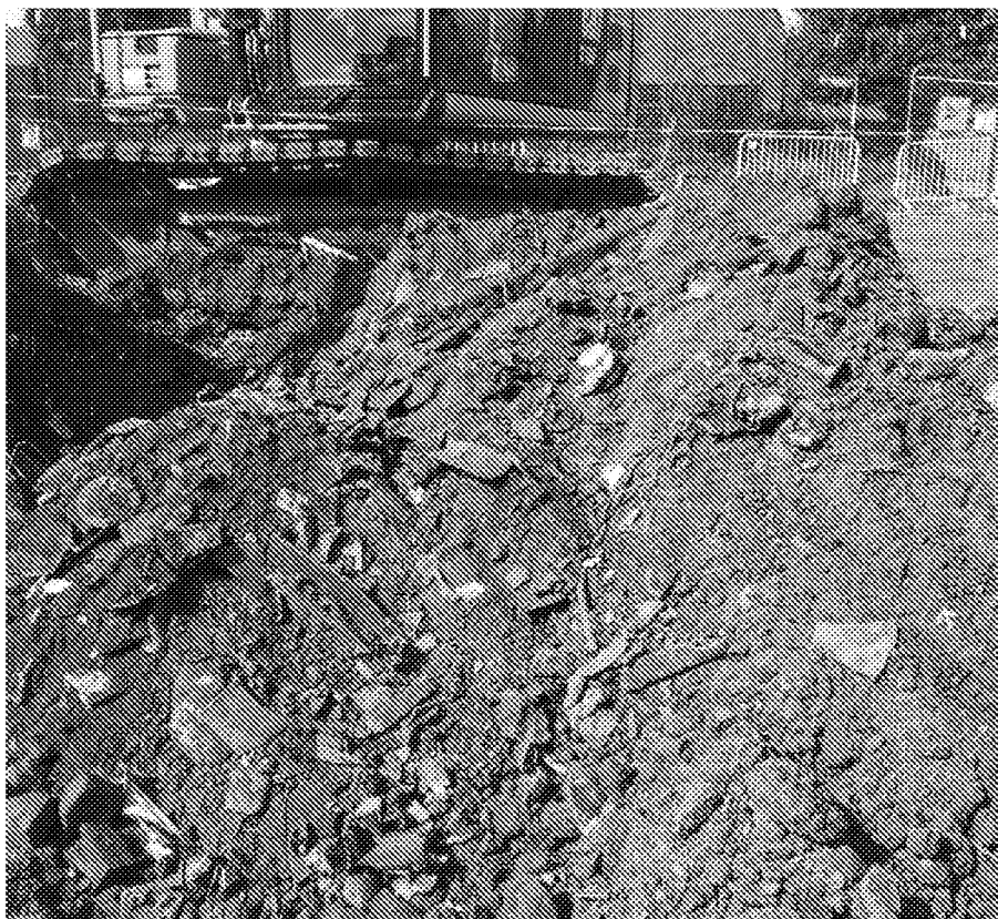
Figure 13: Asbestos removal commences
