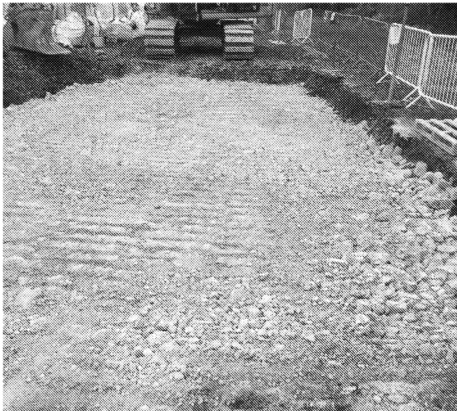
Figure 19: The area is fully backfilled
