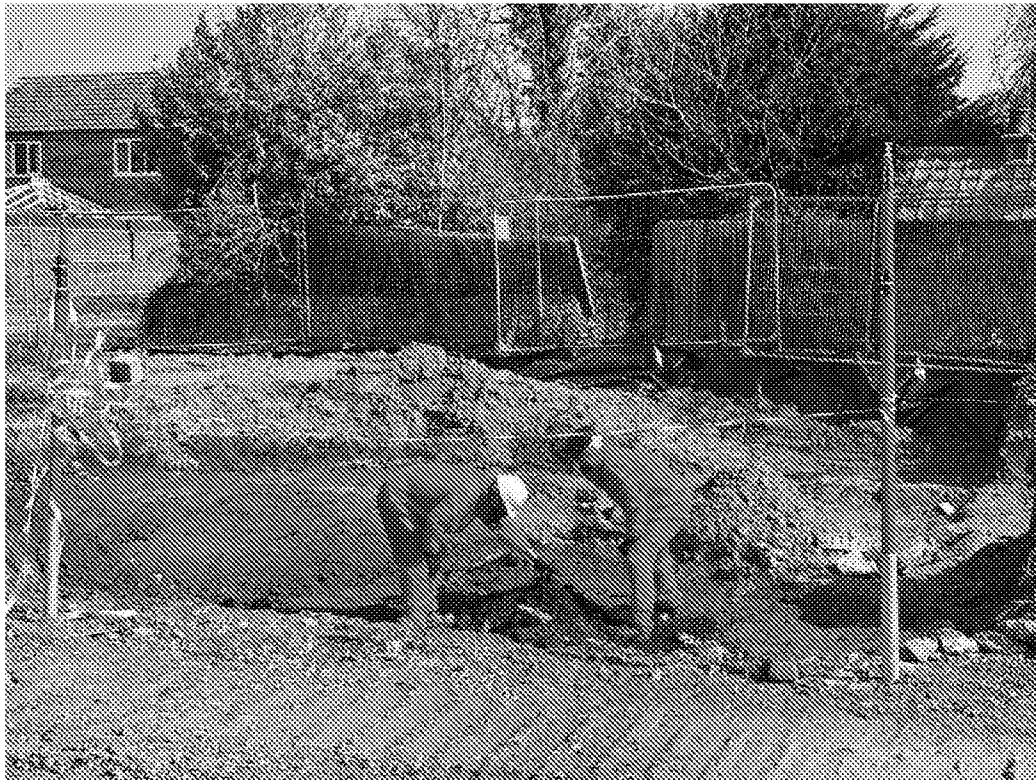
Figure 16: Asbestos contractors locate and dispose of materials
