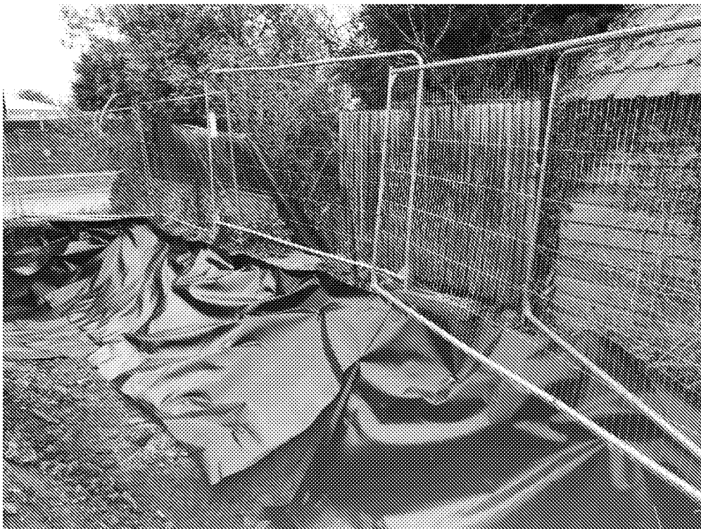
Figure 11: Root barrier membrane installation works
