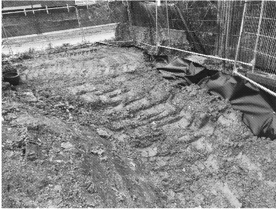
Figure 12: The root barrier membrane is backfilled with clean site won material
