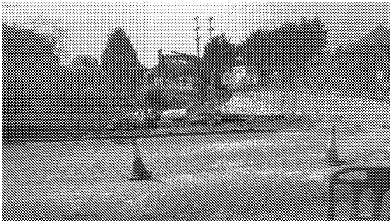
Plate 3 View across the site following the Made Ground excavation
