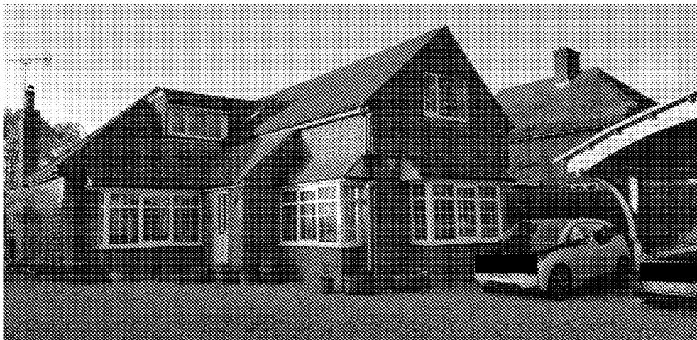
Existing front (East) elevation from approach driveway
