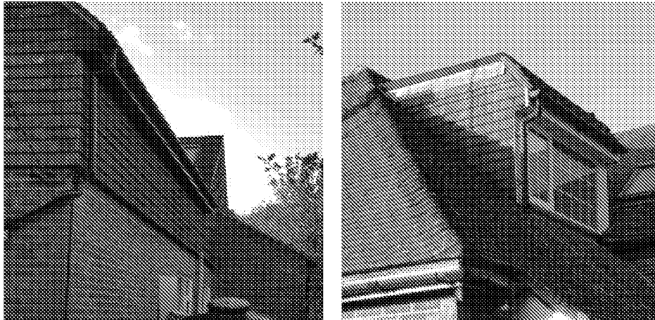
Existing hanging tile (left) and existing front dormer window to Bedroom 4 (right)
