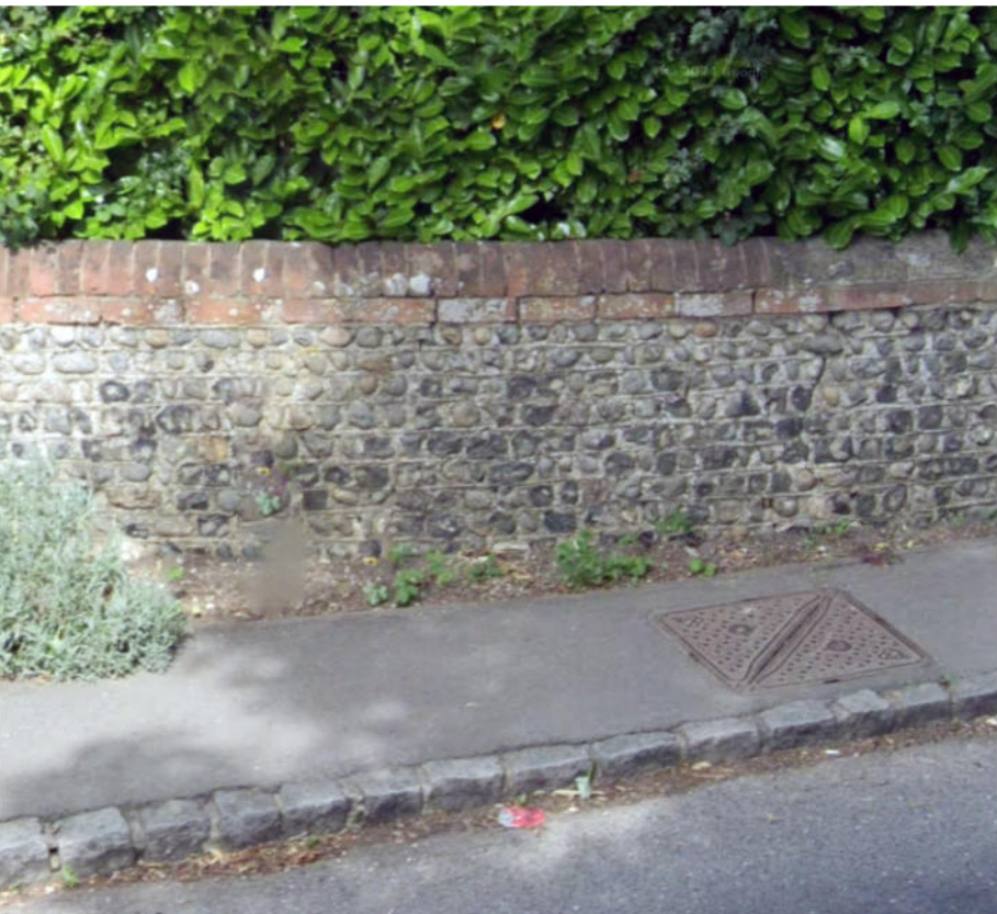
PHOTO OF EXISTING BRICK & FLINT WALL | AS VIEWED NORTH OF APPLICATION SITE
