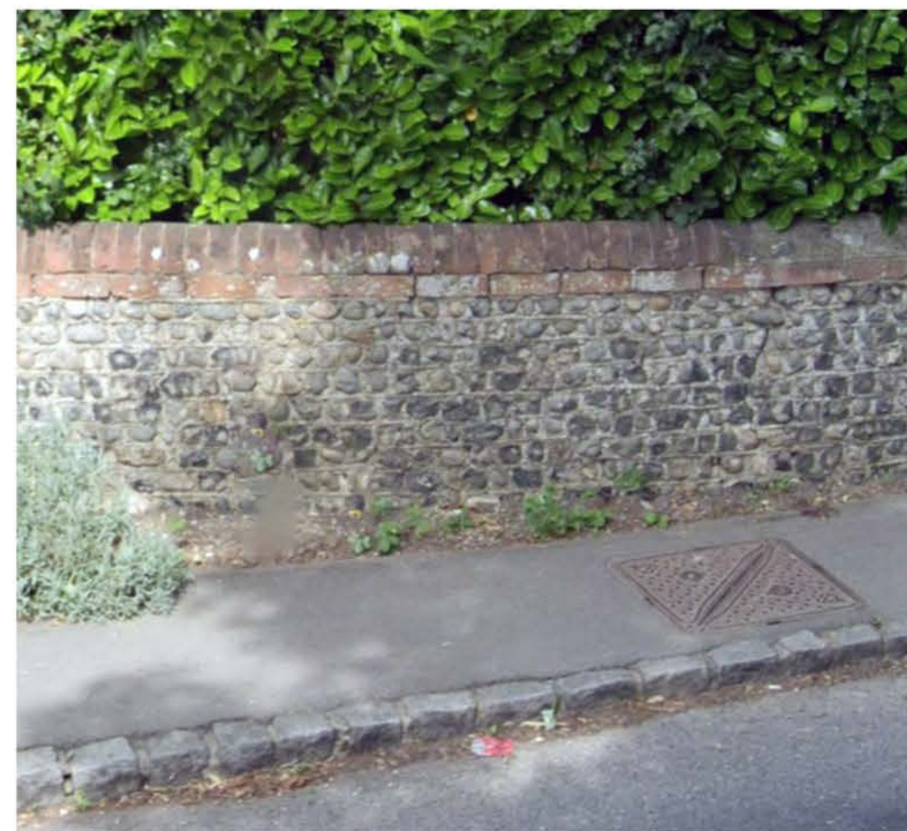
Photograph reproduced from EW601 - wall north of the application site.
