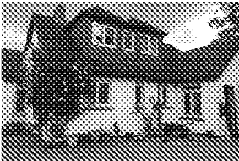
Figure 3. Front elevation of dwelling.
