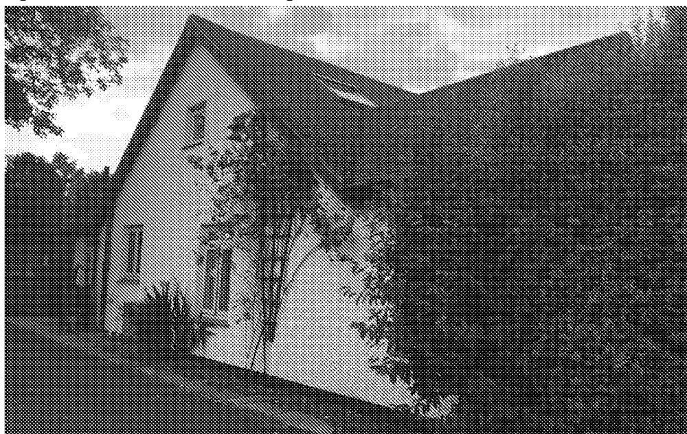
Figure 4. Rear elevation of dwelling.
