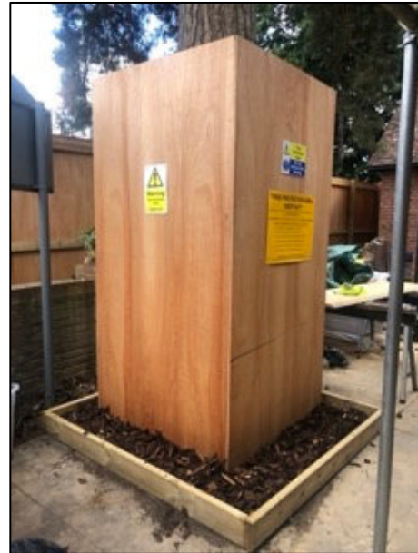
Trunk Protecta® ( GreenGridSystems.com ) & Timber stem protection boxing
