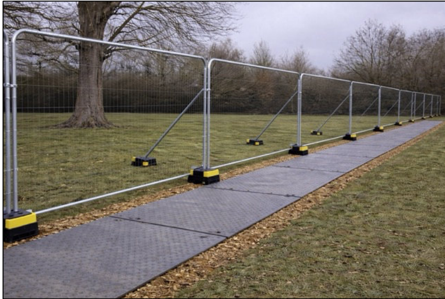
Ground protection example — wood chip and trackmats
